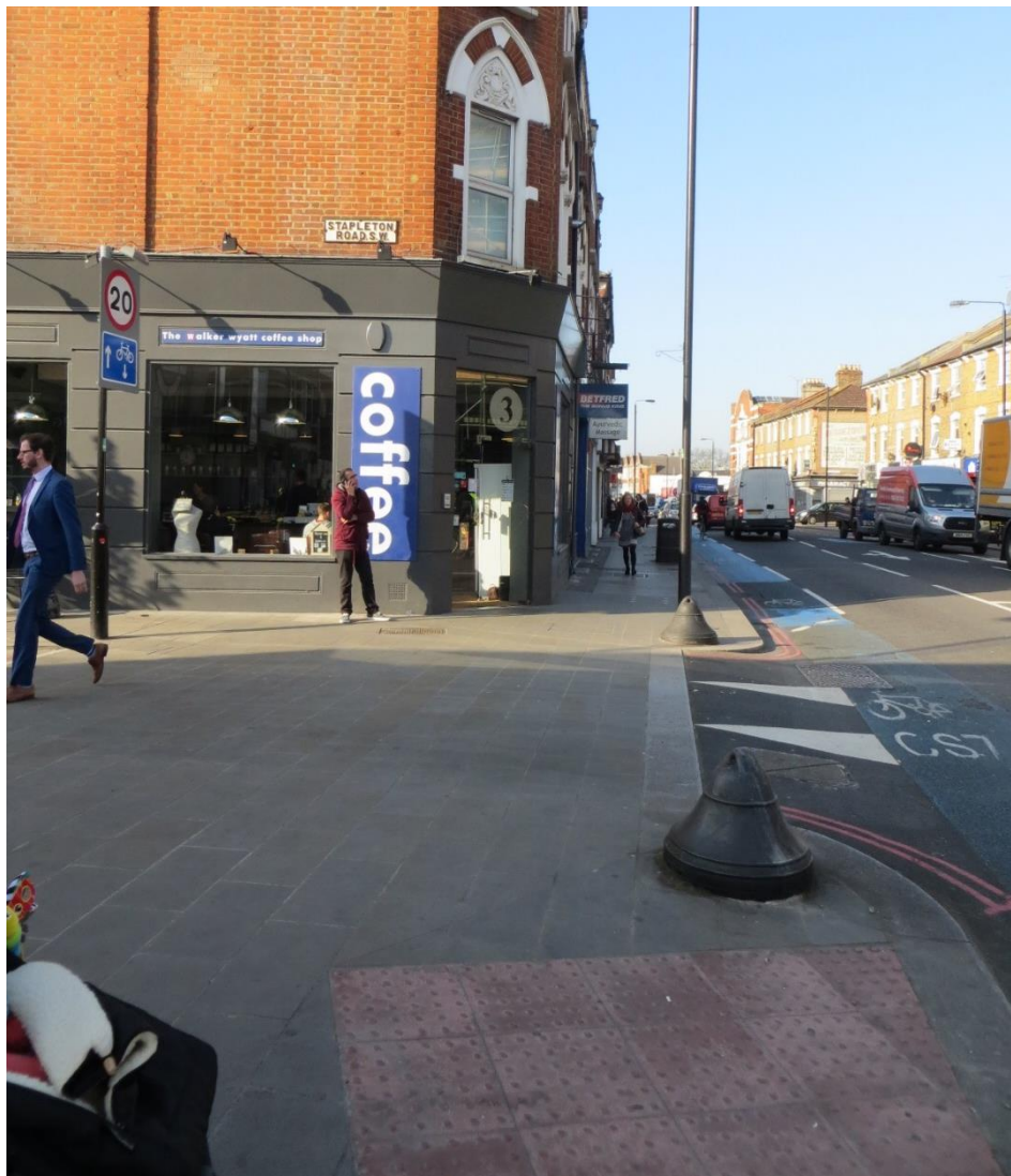
Figure 4.26: Tight corner radius with bell bollard at Site 7
