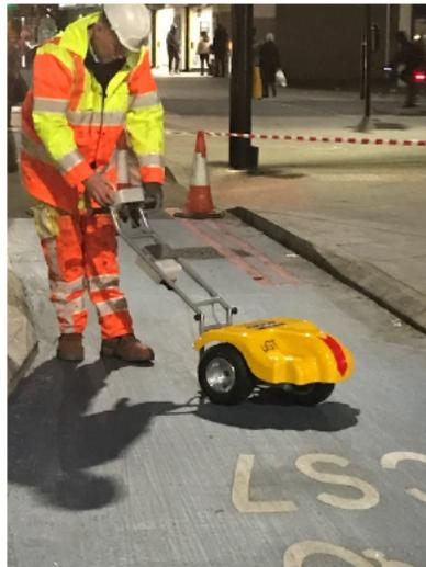
Once Traffic management was installed WJ Operatives investigated the defective areas of MMA cycle lane surface treatment, it was soon discovered the surface course material underneath the MMA surface treatment has been contaminated, causing the cycle lane MMA Surface treatment to fail – crack and lift.
