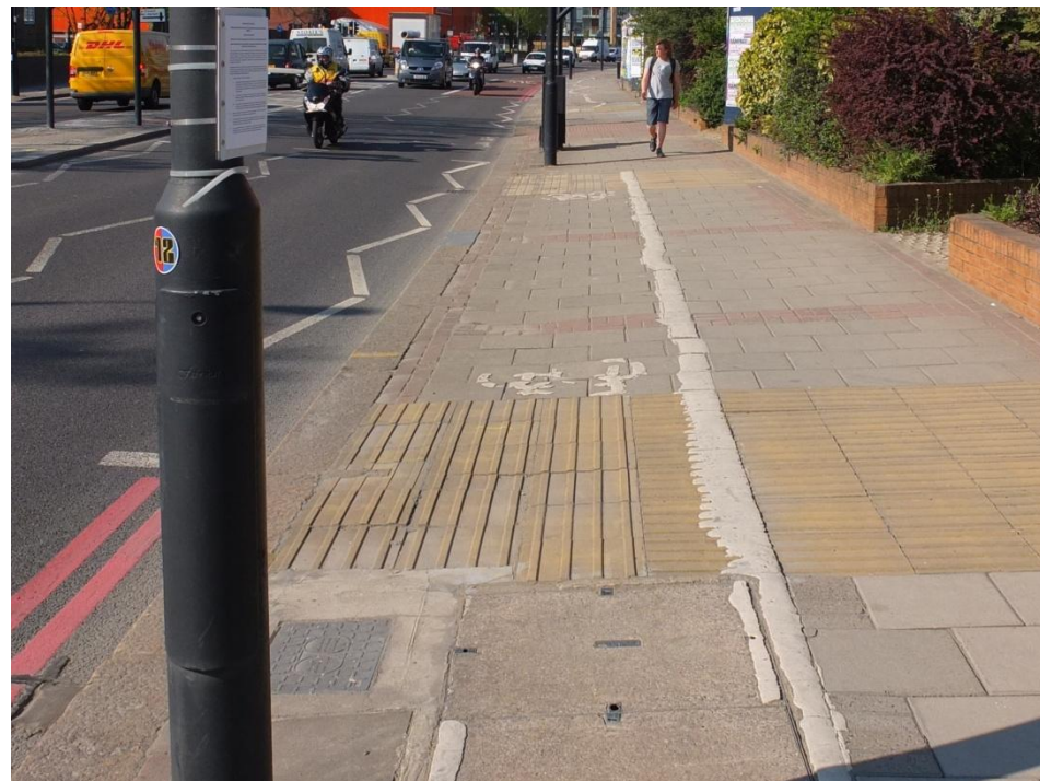
Unsafe/obstructed off-carriageway provision
