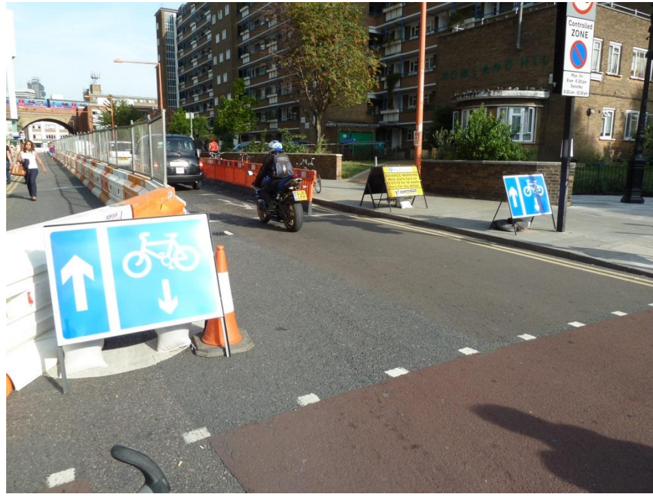
Good treatment at road works
