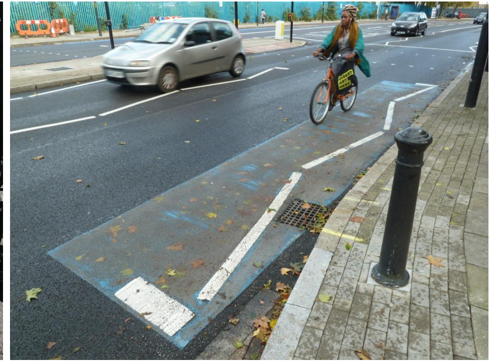
Poorly marked provision
