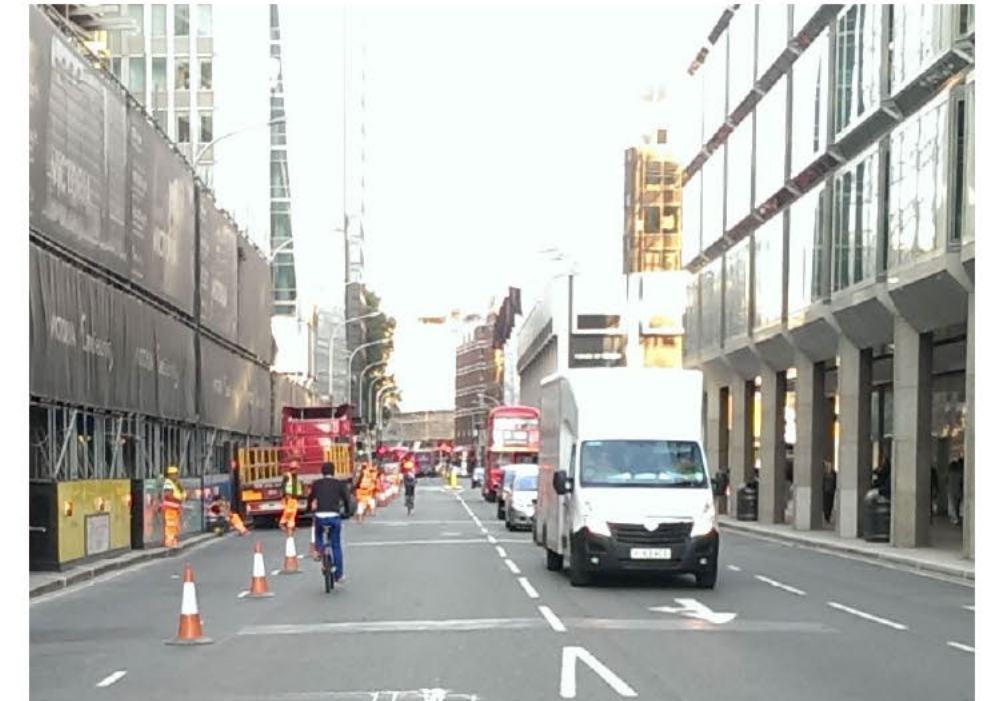
Victoria Street, showing lane closed for construction works
