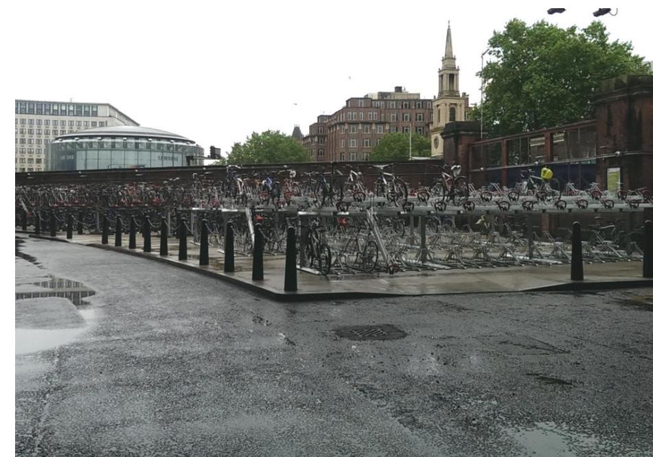
New cycle parking, Waterloo Station
