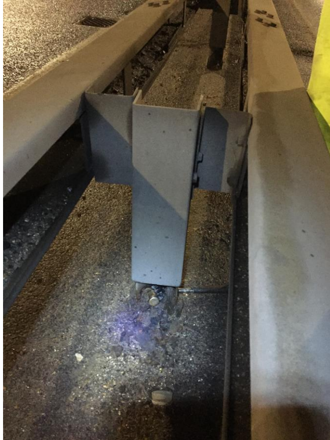
Photo 4 – Perforation of post with mild hammer tapping
