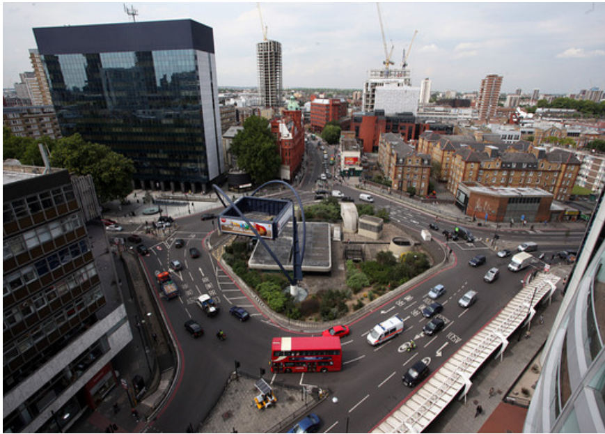
Figure 2: Old Street Roundabout – built environment
