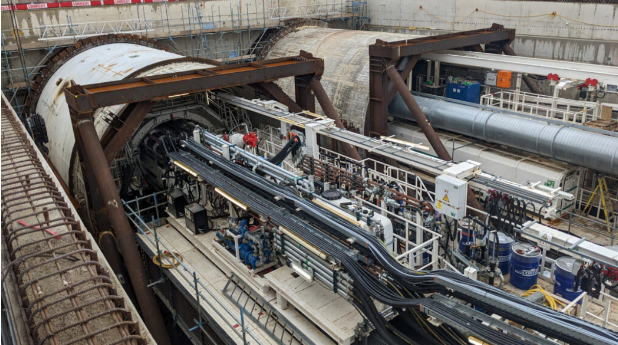
Two HS2 TBMS – at Ruslip earlier this year
