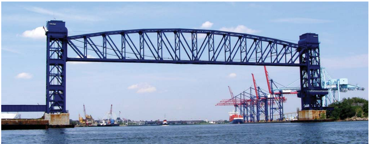
Figure 9 The Arthur Kill lifting railway bridge, new York in the fully open position.
