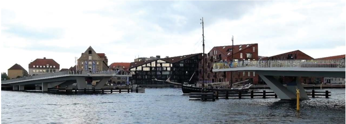
Figure 8 Inner Harbour Bridge, Copenhagen, in the open position to allow a vessel to pass.
