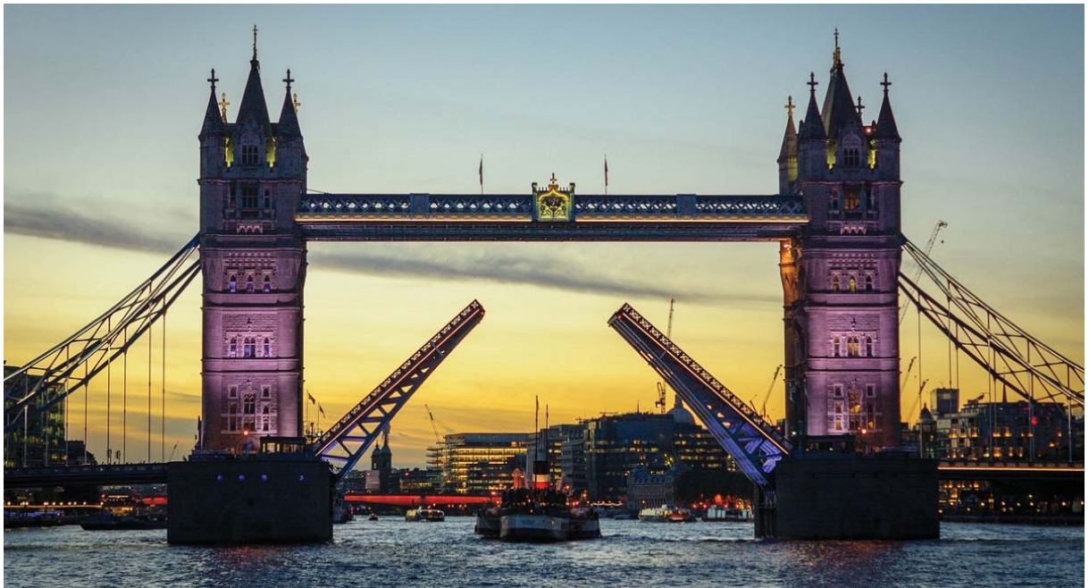
Figure 4 Tower Bridge, London, partially open to allow a medium-sized vessel to pass. A much larger vessel would require the leaves to rotate to almost the vertical position.
