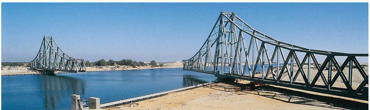
Figure 6 El Ferdan Railway Bridge over the Suez Canal, Egypt, in the half-open position.
