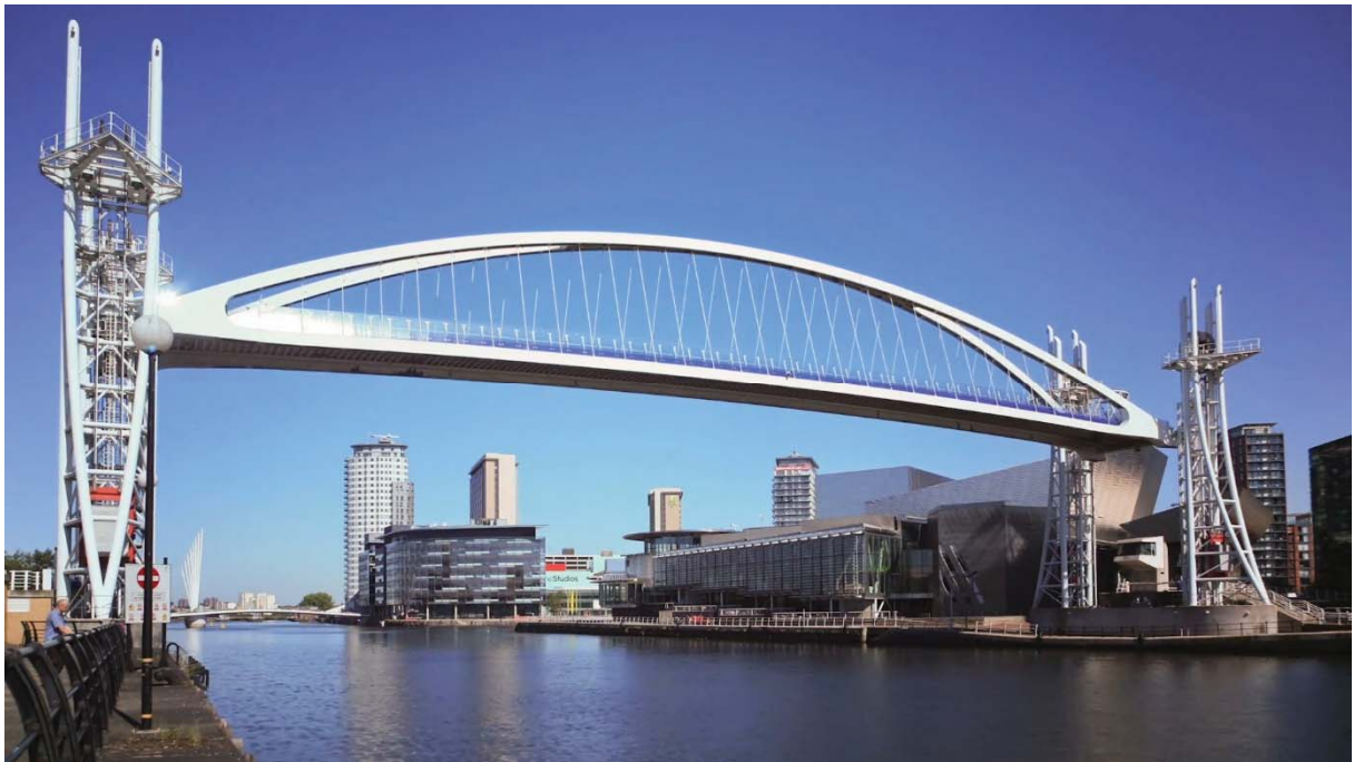
Figure 7 Millennium footbridge at the Lowry Centre, Salford Quays, in the partially lifted position.
