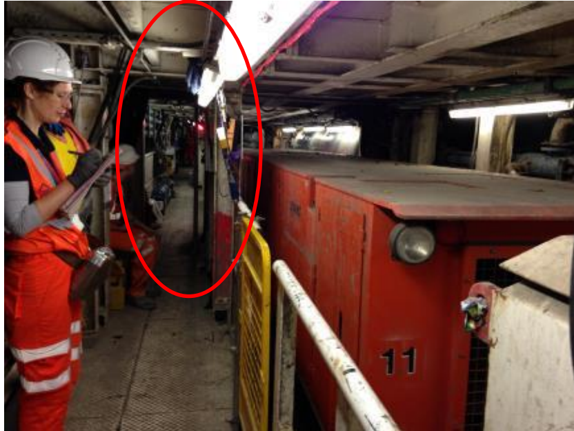
Figure 6: Static samplers at group pump operator station. Figure shows locomotive and grout pump operator (seated). Researcher recording locomotive movements.
