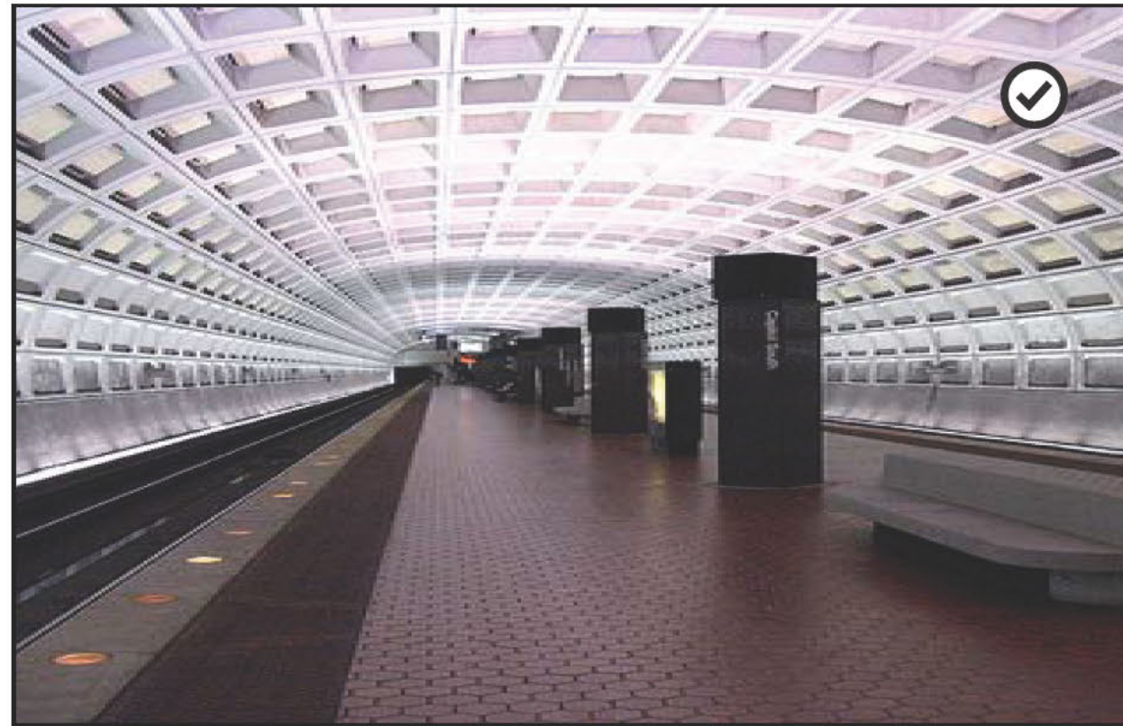
Vertical surfaces opposite platform are illuminated from linear in-ground sources to make the full volume of the space apparent. Indirect lighting from uplights in the totems provides the general illumination.
