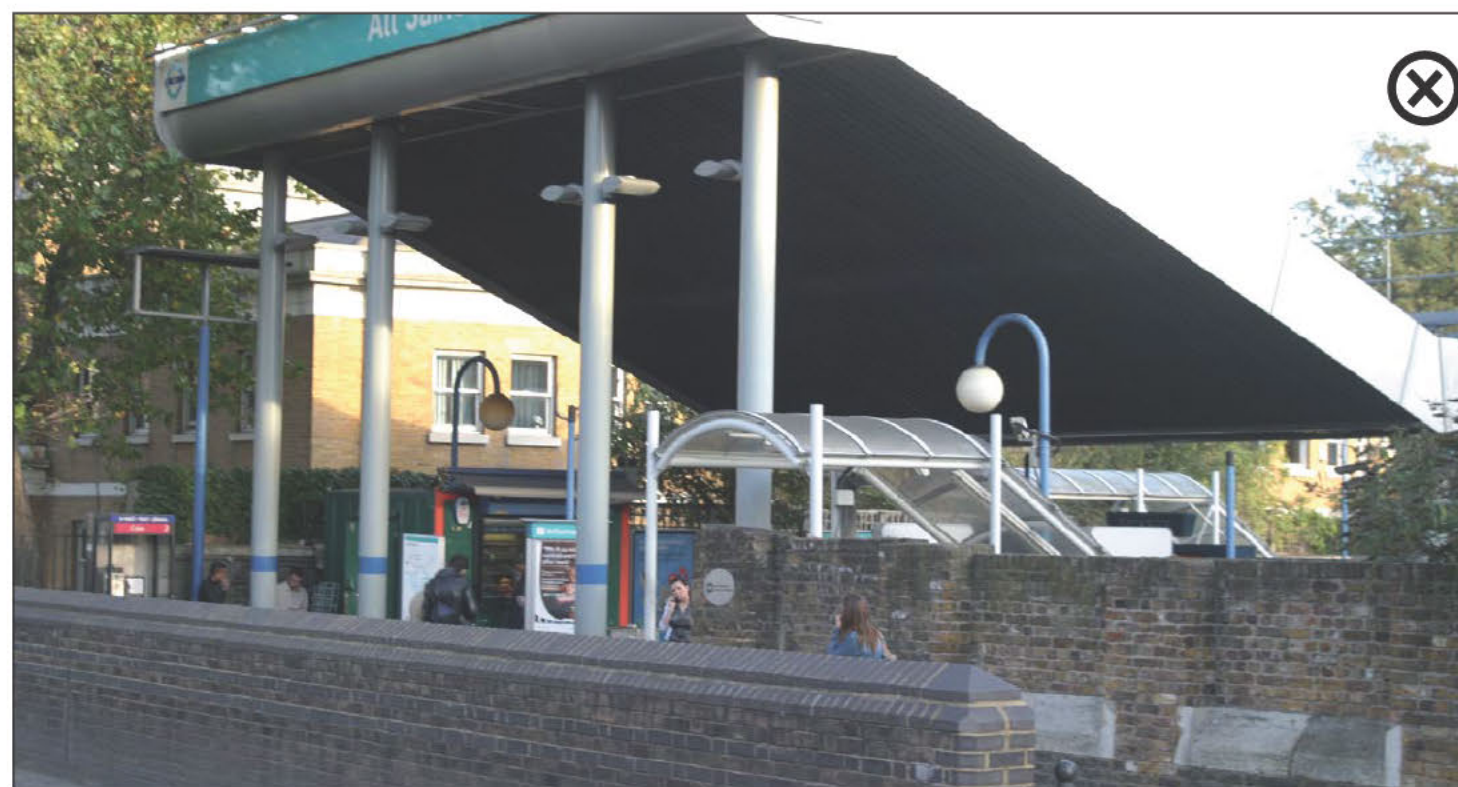
All Saints Station: brick walls and highway parapets obstruct views.
