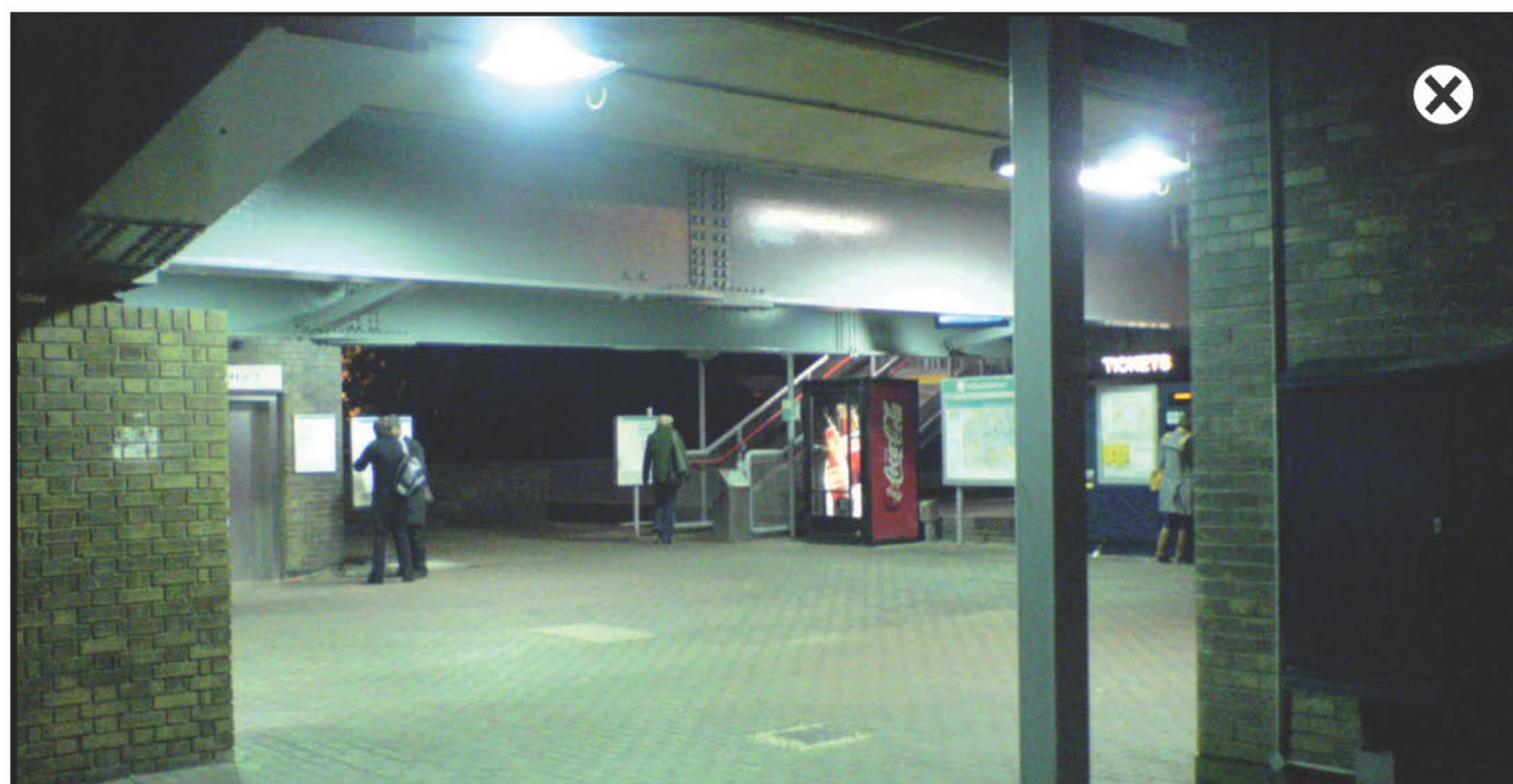
Concourse area lighting is purely functional. There is no highlighting of signs, stairwell or lifts to aid wayfinding.
