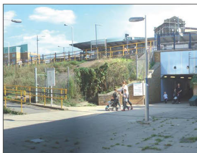
Concourse beside solid viaduct – Greenwich (6.1.5)
