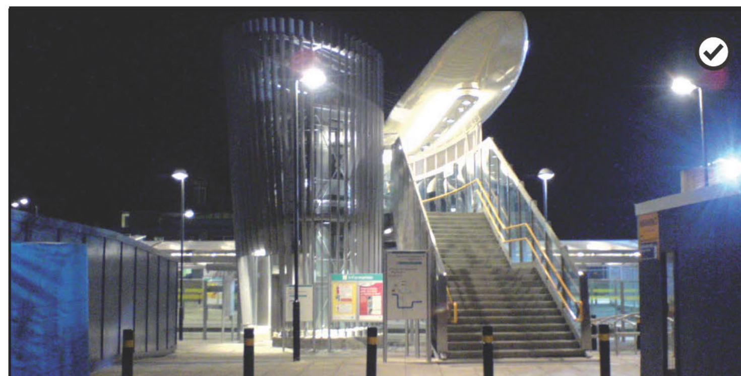
Architectural form with integrated lighting clearly defines routes; lighting columns are located at the edges of the space to maintain views.
