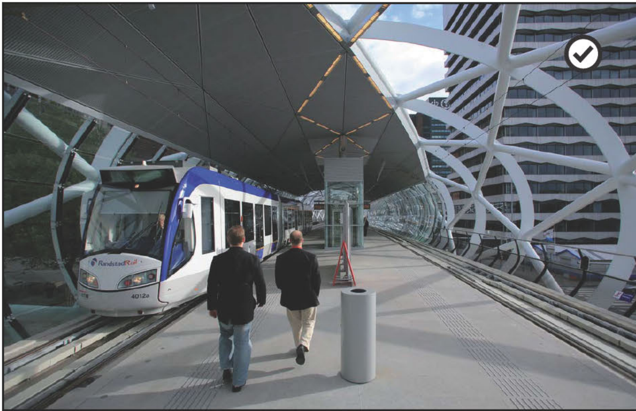
Platform lighting is integrated into the canopy and is louvred to limit glare.
