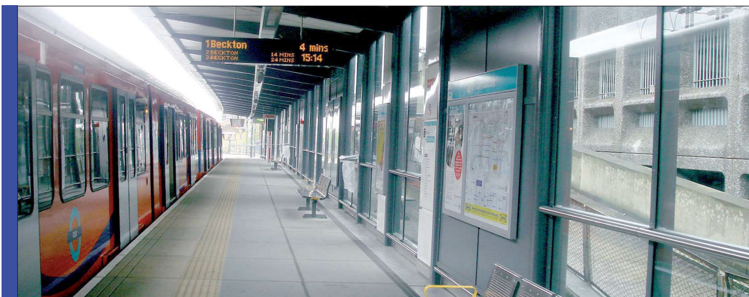
Canopy Replacements (2009). Tower Gateway station
