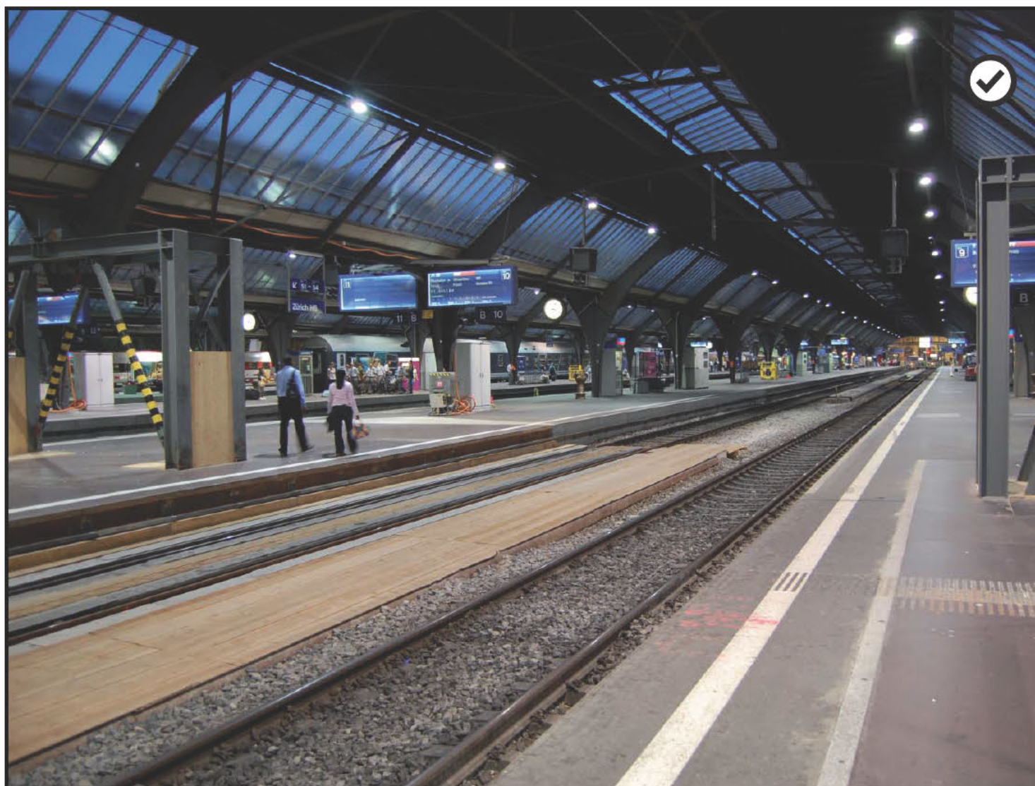
The use of natural daylight should be considered on all new DLR stations and utilised where possible.
