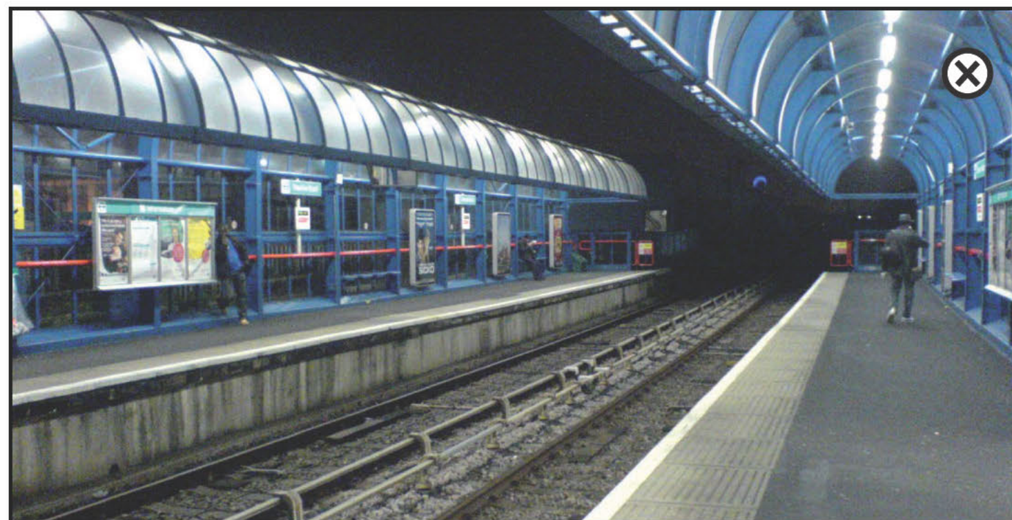
Basic provision only. Surface mounted lighting with no optical control draws attention to the luminaires, are a cause of glare and light pollution
