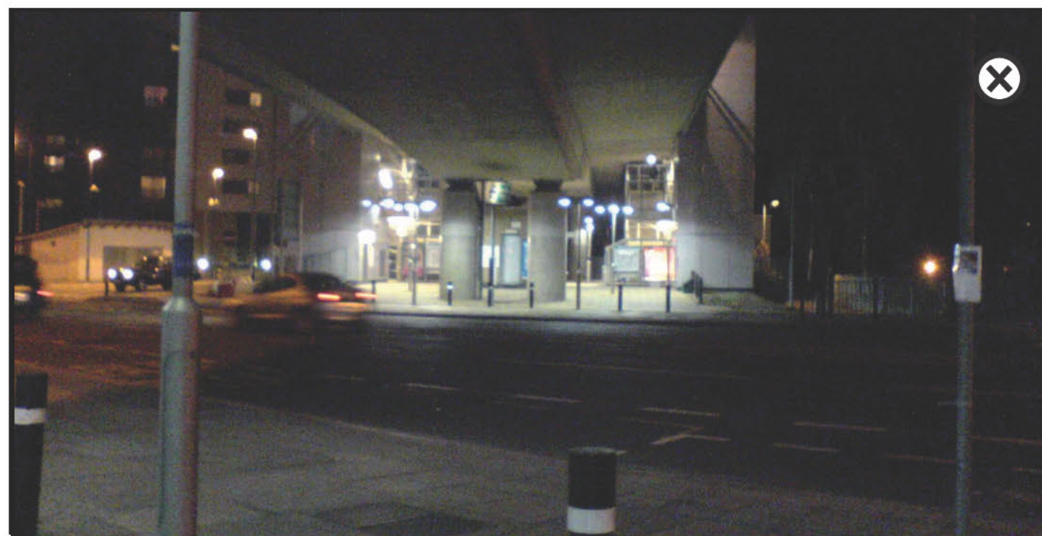
Poor streetscape but station does not integrate subtly into surroundings. Numerous scattered poles leads to cluttered entrance with poor wayfinding. No feature lighting leads to no station identity or character.
