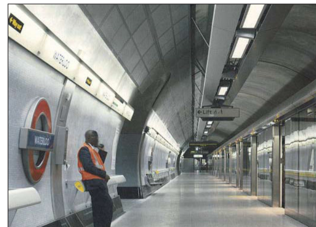
Waterloo station platform: common fixtures
