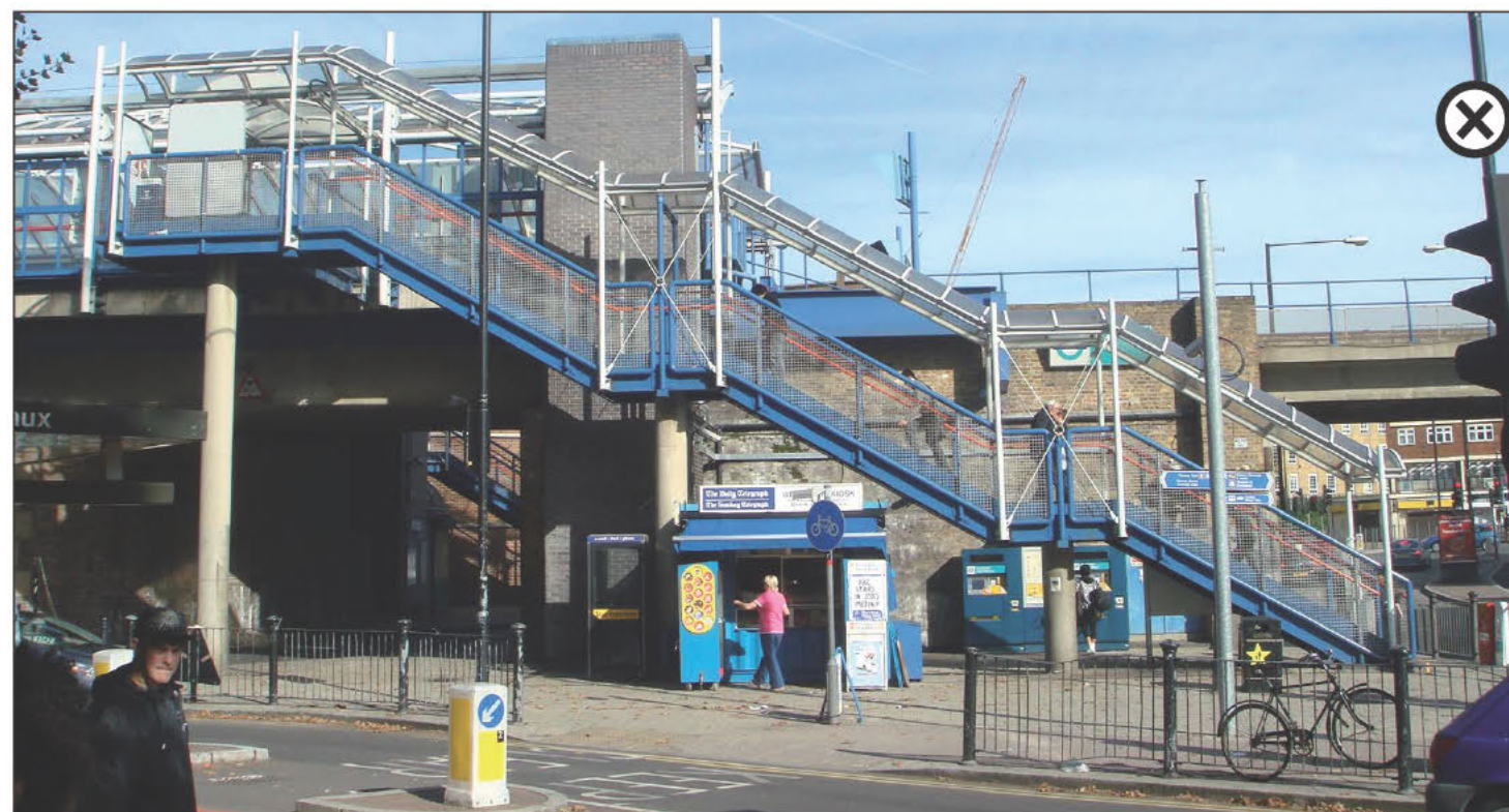
Westferry Station: forecourt has cluttered street furniture and there are many blind corners.
