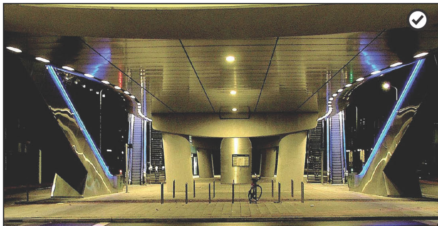
The use of coloured lighting and increased illumination levels to highlight the escalator entrance to the station.
