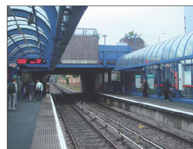
Concourse above cutting – Devons Road (6.1.6)
