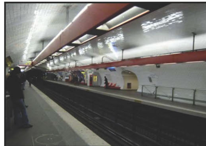
Ceiling of station with ceramic tiles, the fitting is reflected in the material.
