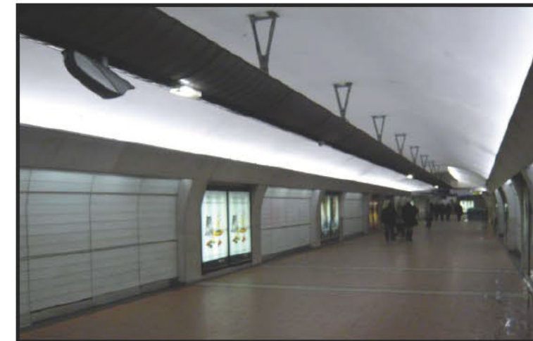
Concrete ceiling used as a reflector for a diffuse lighting.
