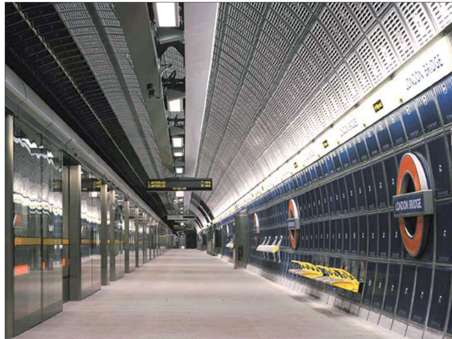
London Bridge station uses similar cladding to other stations and common fixtures such as seats, boom and frieze
