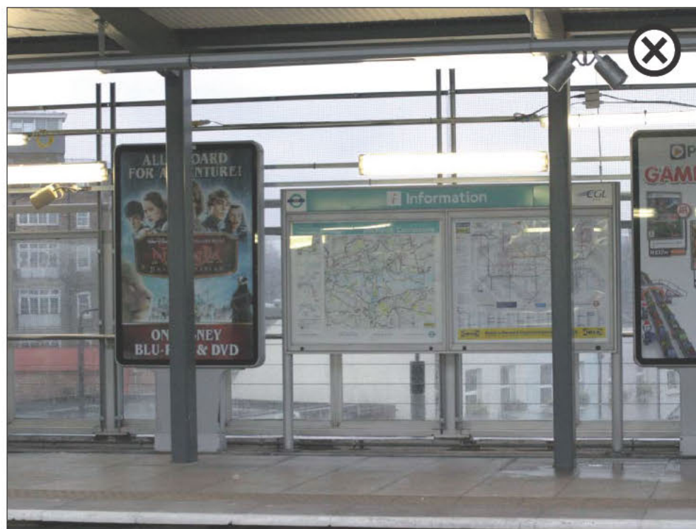
Deptford Bridge DLR Station: lack of coordination of elements on the platform
