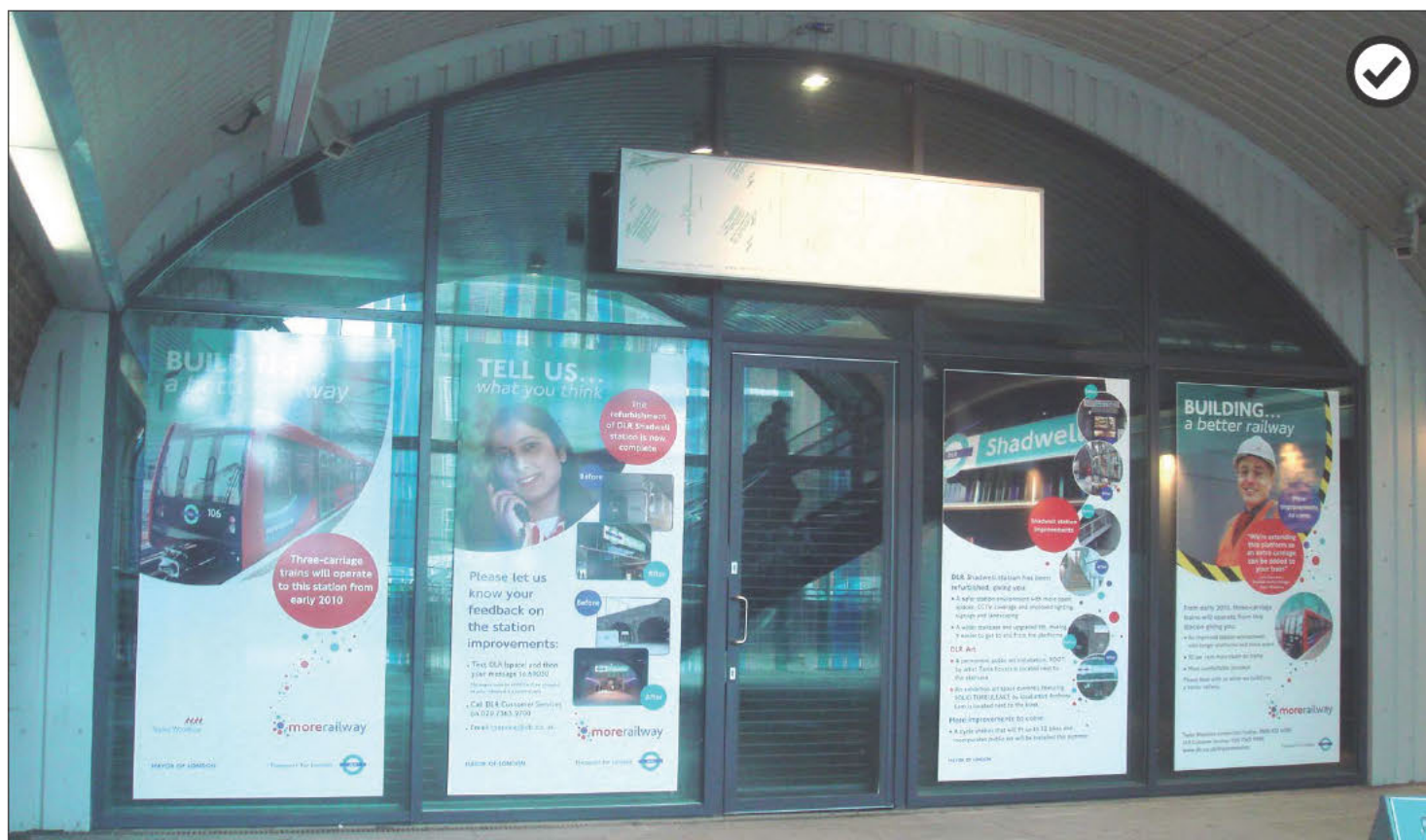
Existing viaduct arches used as retail units at Shadwell station
