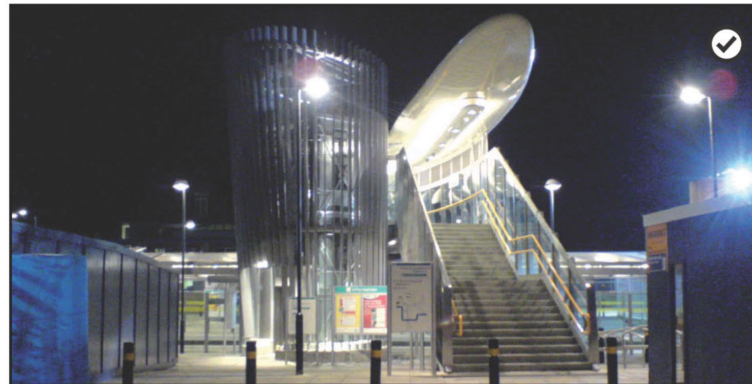
Base lighting provides good illumination levels and colour rendering makes the space both safe for functional use and provides a feeling of security.
