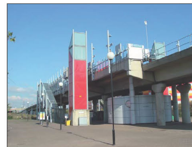
Concourse under viaduct – Gallions Reach (6.1.4)
