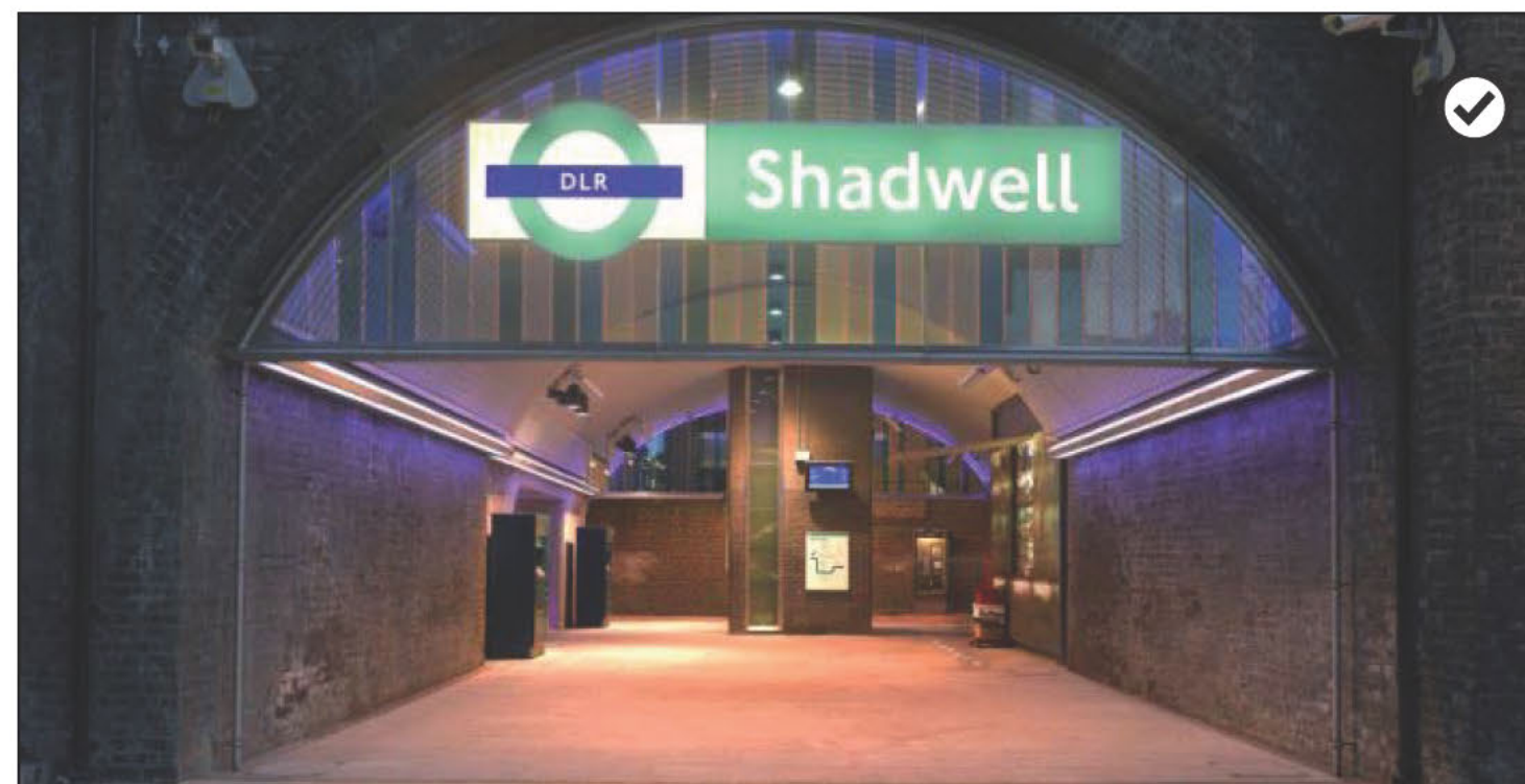
Well lit archway with good illumination levels and coloured lighting accentuating viaduct structure and providing a degree of interest
