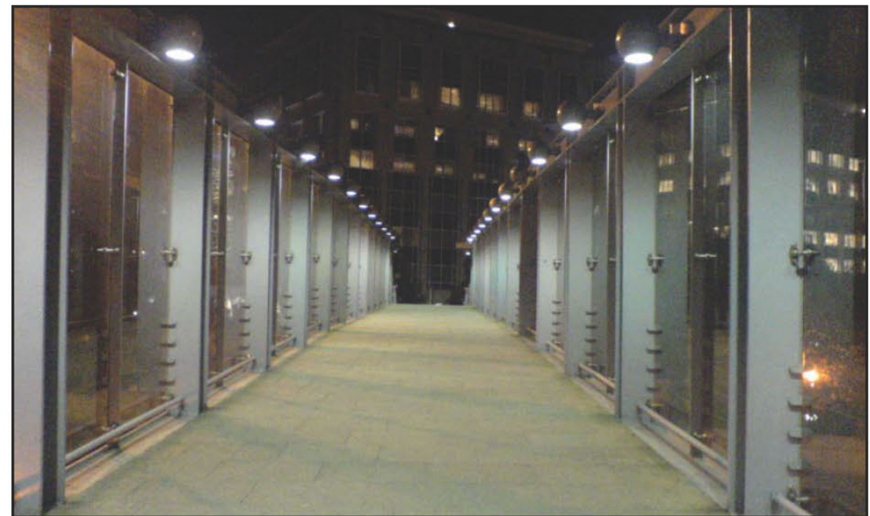
Luminaires with a controlled optic allow for good level of illumination without inter-reflection the glass allowing for a view into and out of the bridge.
