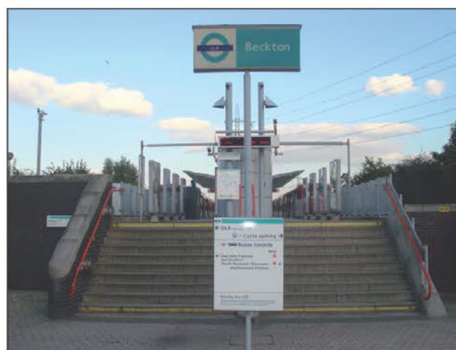
Concourse at end of platform – e.g. Beckton (6.1.3)
