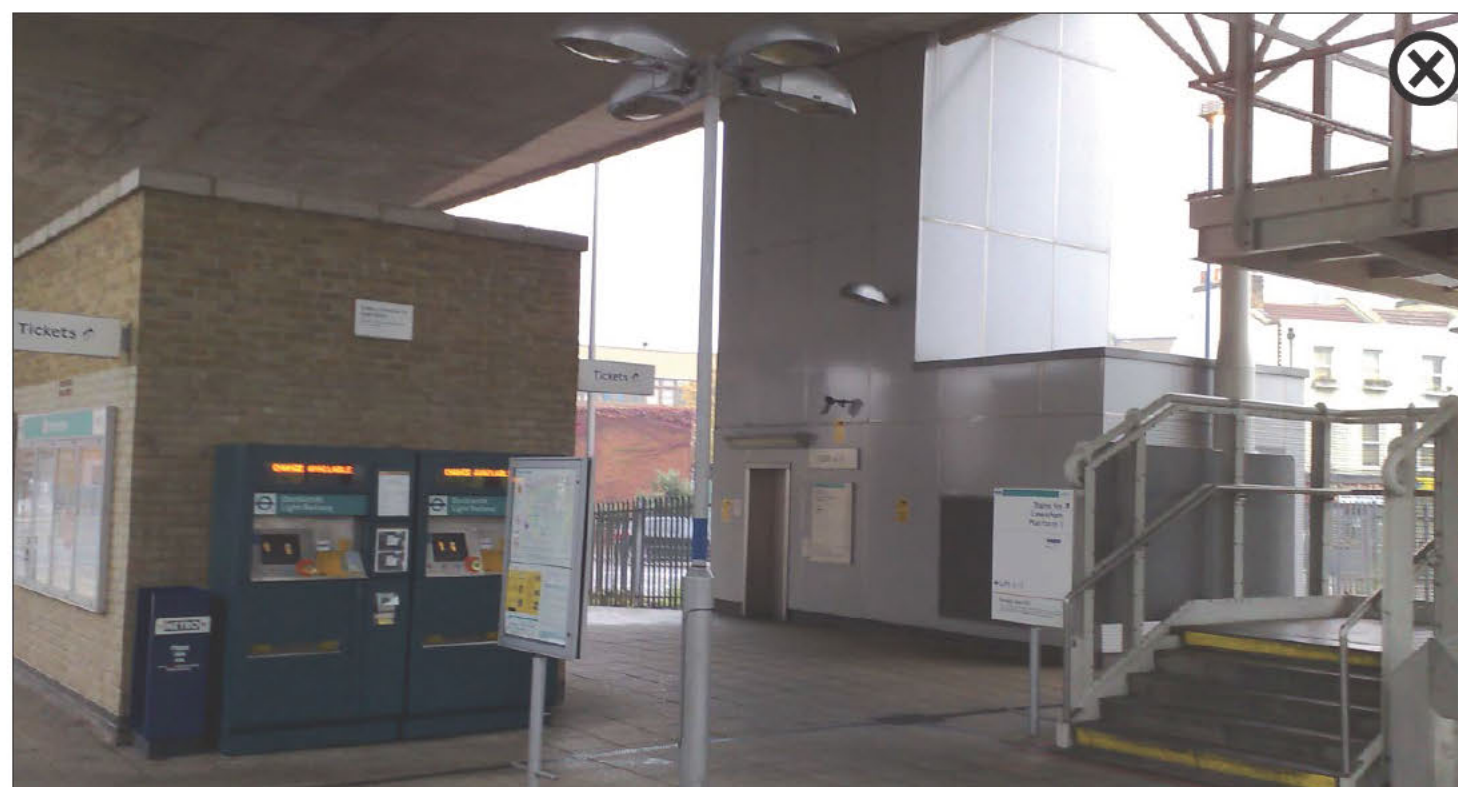
Deptford Bridge Station – Information and ticket vending machines are scattered around the concourse making them difficult to find.
