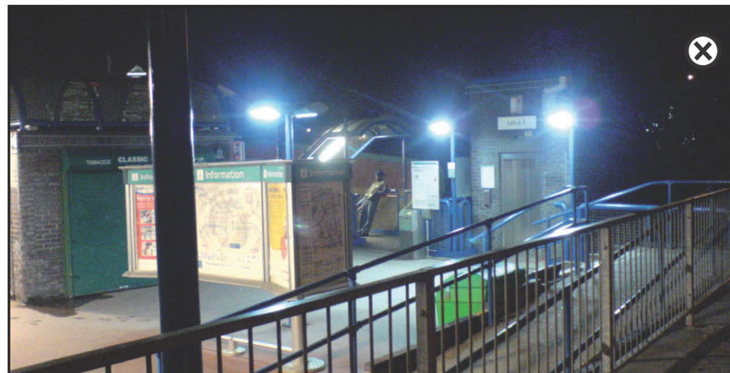
Basic lighting columns which visually clutter the space, and with visible lamp sources which disrupt views and are a source of glare.
