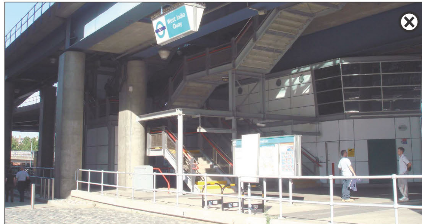
West India Quay station has awkward entrances and layout which prevent direct routes to information, ticket machines and platforms
