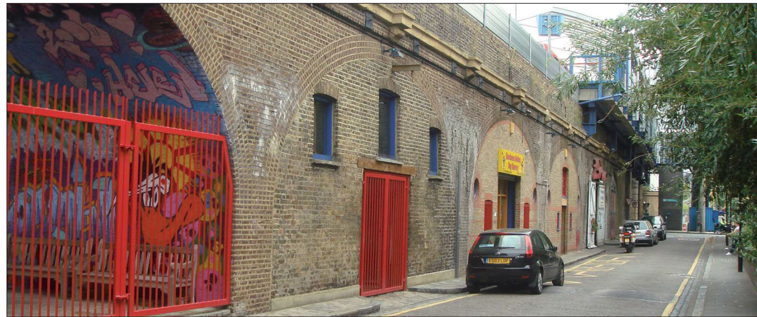
Solid/Vaulted Viaduct – Westferry (8.1.3)
