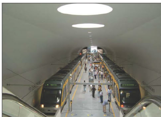
An Island Platform on Porto Metro shows a controlled palette
