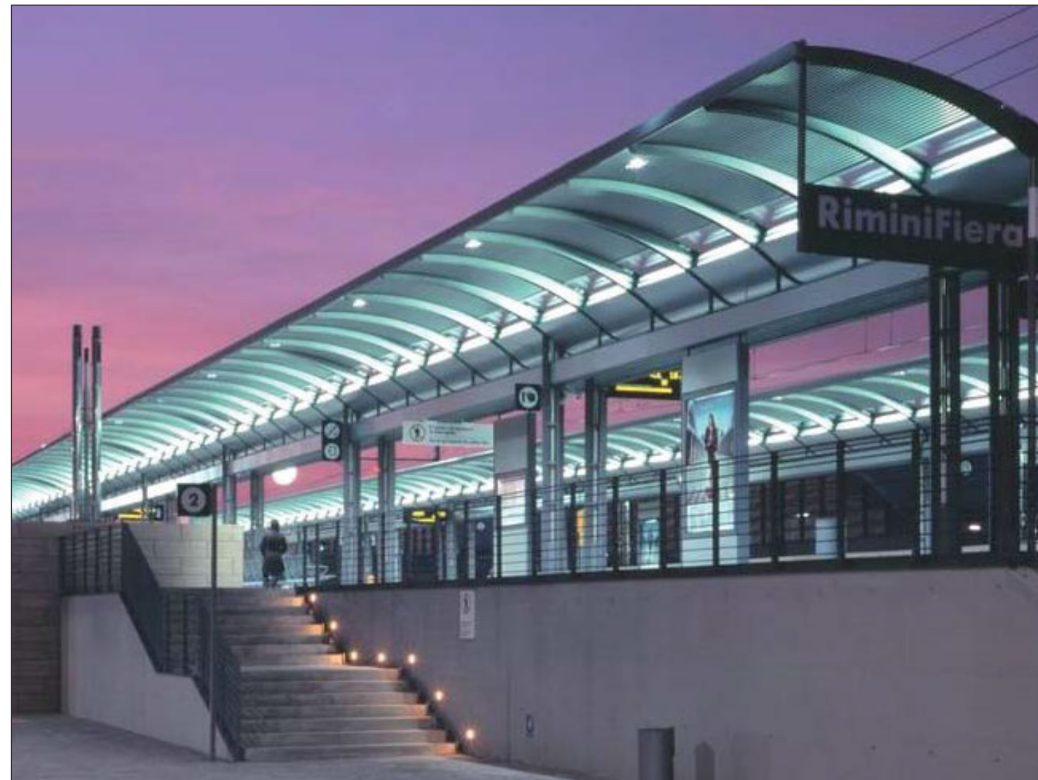
Rimini Station in Italy uses a Deutsche Bahn canopy
