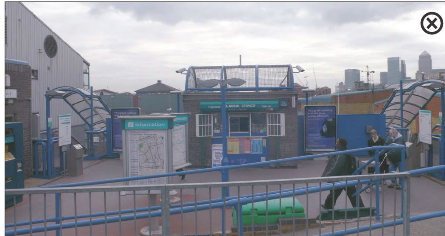
Devons Road concourse is difficult to navigate and has poor visibility due to extensive clutter and lack of visual hierarchy.
