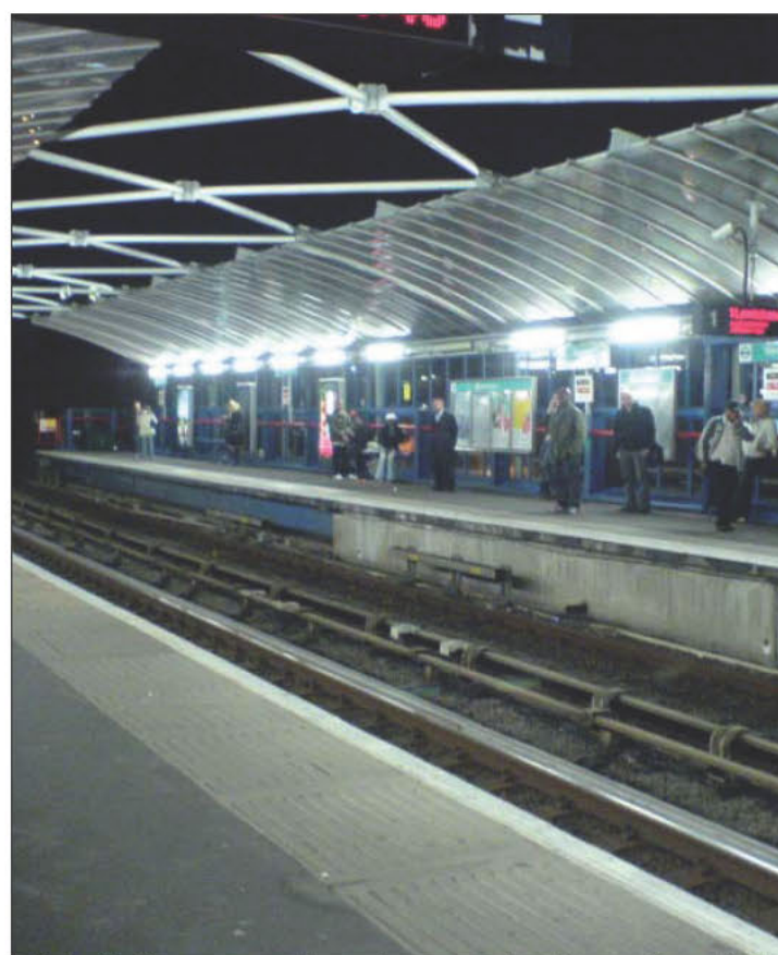
Unshielded luminaires resulting in large porportion of upward loss of light
