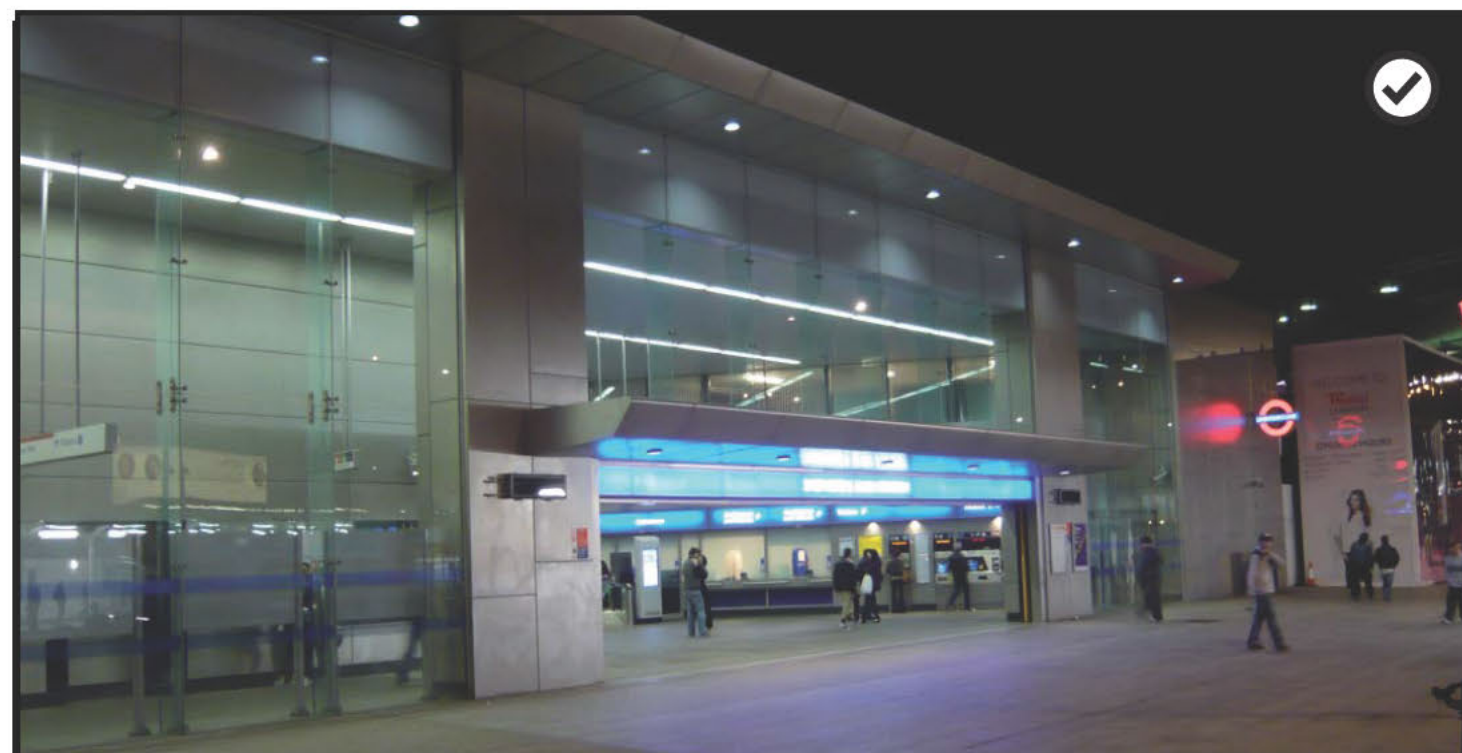
Safe illumination levels, good signage, integrated lighting to reduce clutter and coloured lighting helps to give the station identity.
