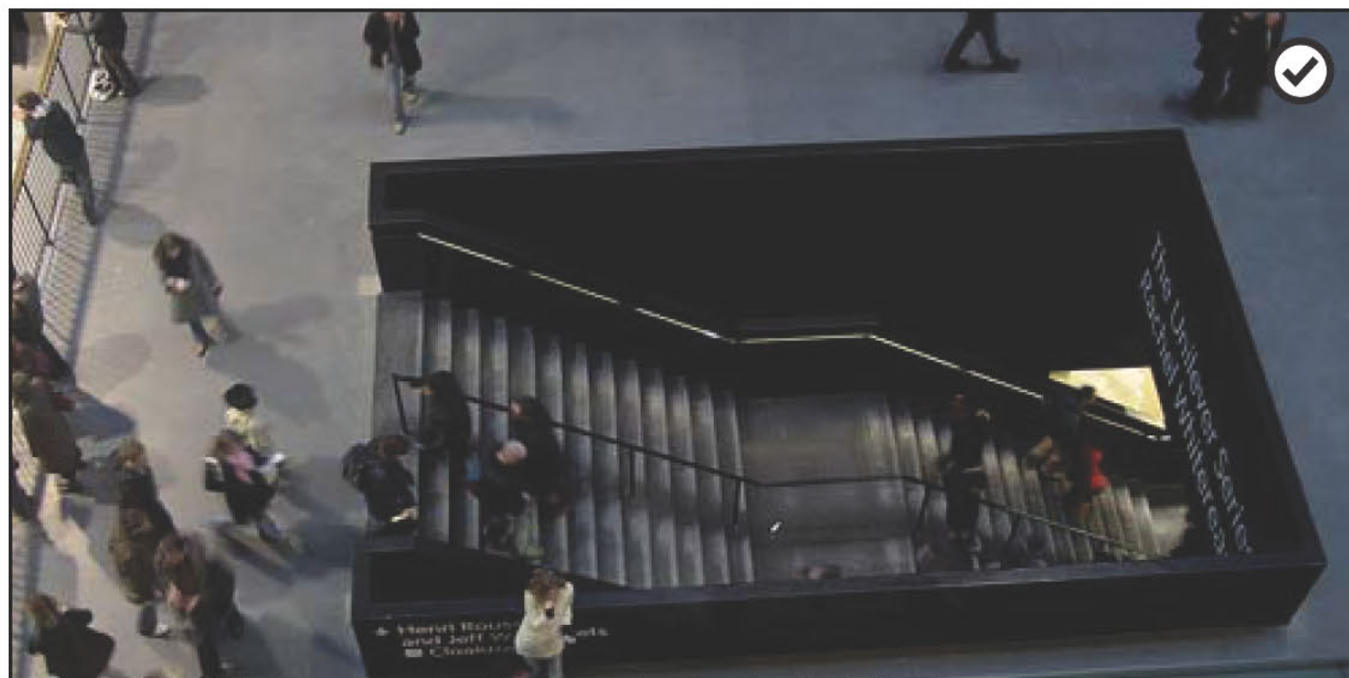
Lighting integrated into the handrail provides a guide as to the stair geometry and provides ambient lighting to the space.
