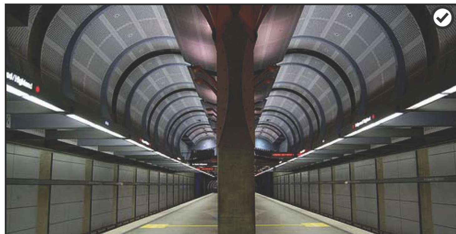
Feature uplighting of ceiling highlights its unusual shape, texture and provides a sense of volume to the space. Illumination of wall surfaces provides for a balanced visual field.
