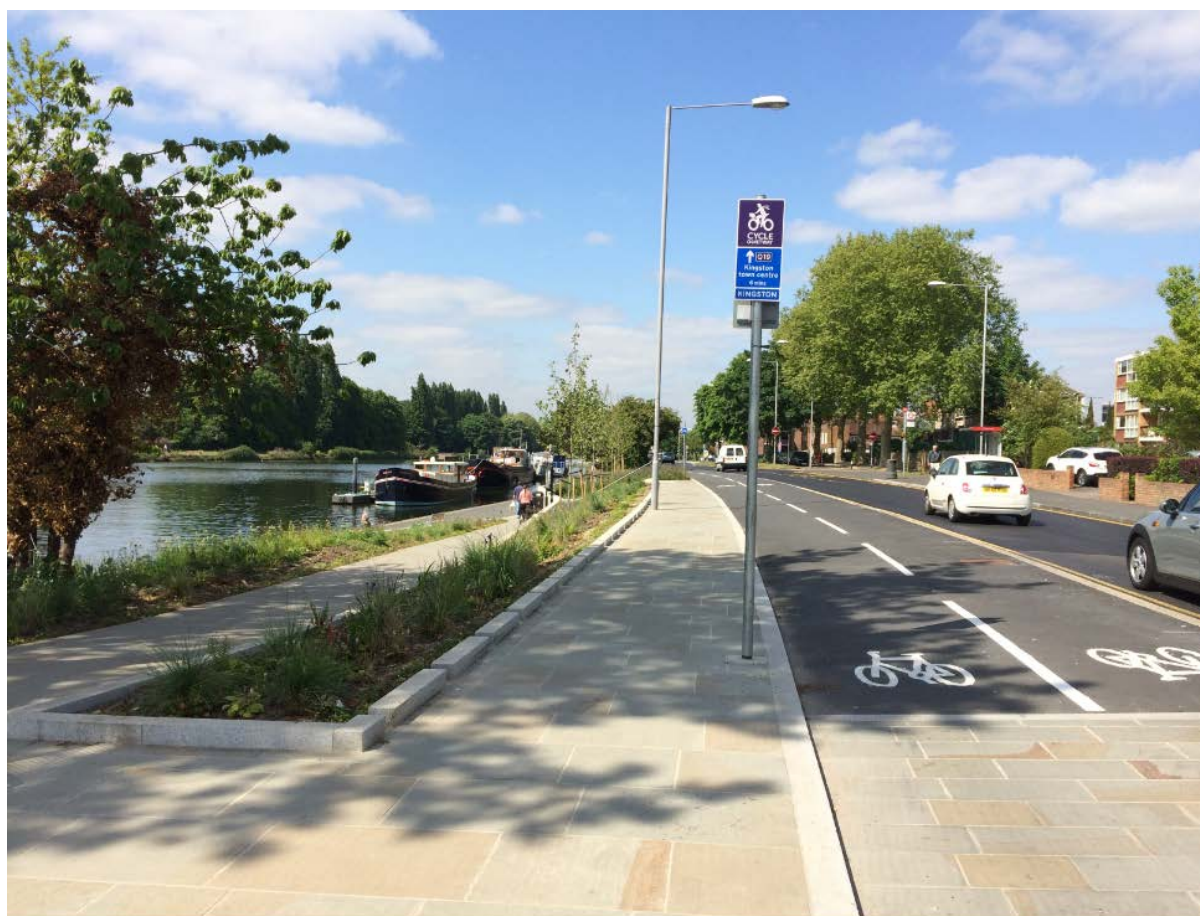
Figure 5.27 Portsmouth Road, Kingston – showing the new two-way cycle lane.
