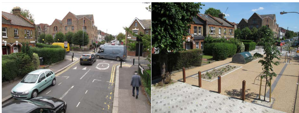
Figure 5.26 Example of a filtered permeability scheme at a junction in Blackhorse Village, Waltham Forest – before and after.
