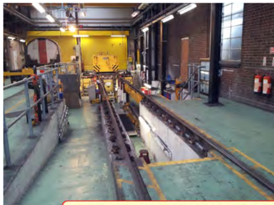
The existing single Headed Wheel Lathe at Northfields Depot on the Piccadilly line
