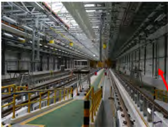
Example Cross Section of a typical modern "Swimming Pool Pit Facility provides improved access to the underframe and side of the train below solebar and increased working space between trains
