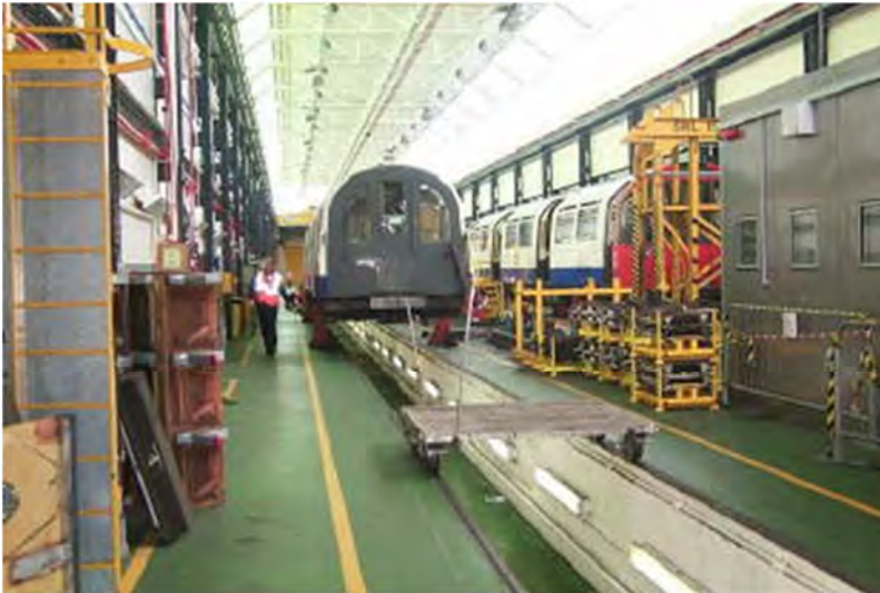
Existing Heavy Maintenance Facility at Cockfosters Depot with a single car lifted on Car Stands and bogie removed
