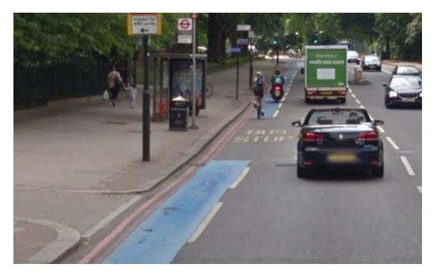
Designing for cyclists on-carriageway around bus stops Where cyclists are on-carriageway, it is important that they are clearly visible to bus drivers, particularly around bus stops. Ideally, cyclists should be able to pass a stopped bus without having to move across into the adjacent lane.
