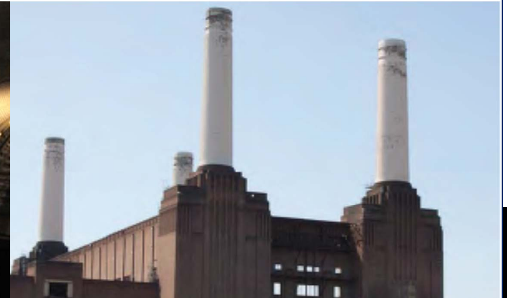
The Northern Line Extension to Battersea, Night Tube, Tottenham Court Road and Camden Town capacity schemes and Fit for the Future - Stations to transform customer experience
