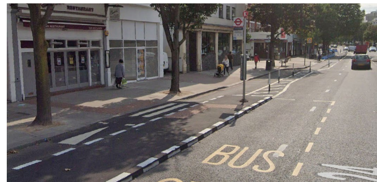
After - Temporary Streetspace bus stop bypass
