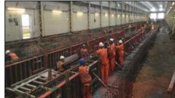
Installation of new pits and platforms
