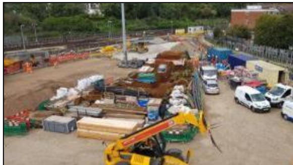
Track fan demolished and site set up
