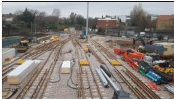
New track installation across all sheds
