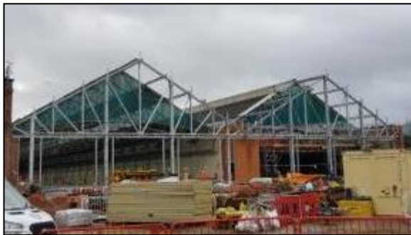
Installation of new gable wall steelwork
