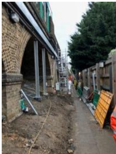
159 pile retaining structure at Barking SER
