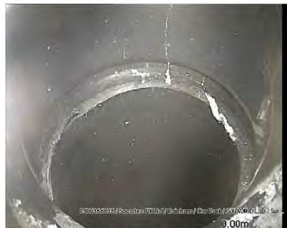
200318_1418D-Survey.jpg, 00:00:08, 0.00 m Line deviates down
