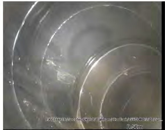
200318_1135F-Survey.jpg, 00:00:11, 0.50 m Line deviates right
