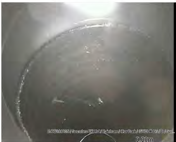
200318_1135E-Survey.jpg, 00:00:04, 0.00 m Line deviates down
