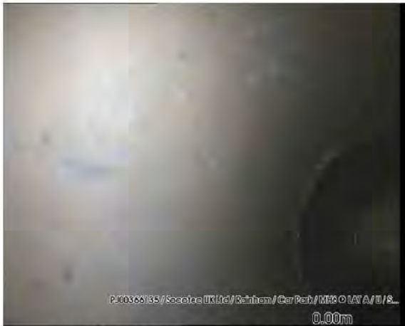
200317_1202C-Survey.jpg, 00:00:00, 0.00 m Start node type, manhole, reference number: MH6
