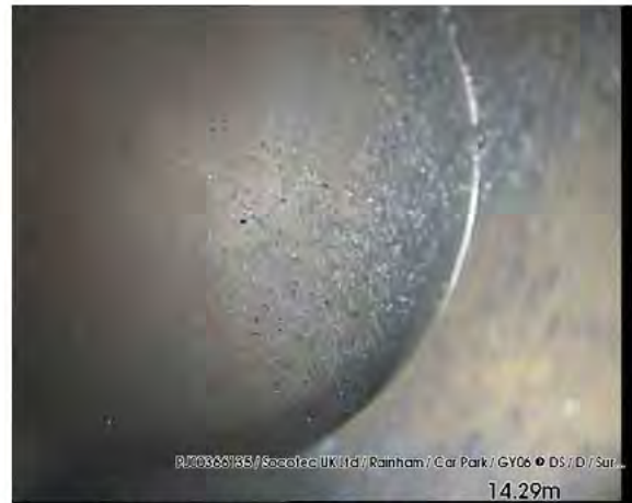
200318_1357A-Survey.jpg, 00:01:44, 14.29 m Finish node type, other special chamber, reference number: DS, interceptor
