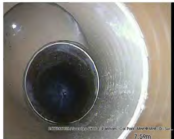
200317_1232C-Survey.jpg, 00:00:25, 7.59 m Junction, at 10 o'clock, diameter: 150 mm
