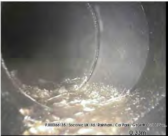
200318_1145A-Survey.jpg, 00:00:10, 0.33 m Line deviates left
