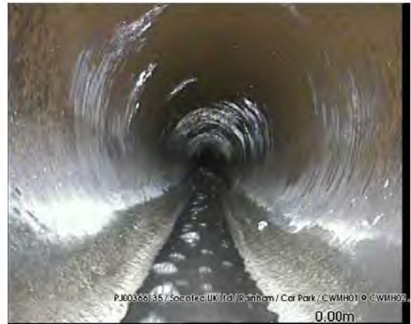
200317_1456D-Survey.jpg, 00:00:02, 0.00 m Water level, 5% % of the vertical dimension, Strong flow
