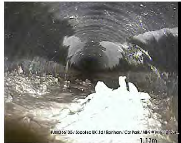
200317_1438A-Survey.jpg, 00:02:08, 1.13 m Survey abandoned, unable to pass
