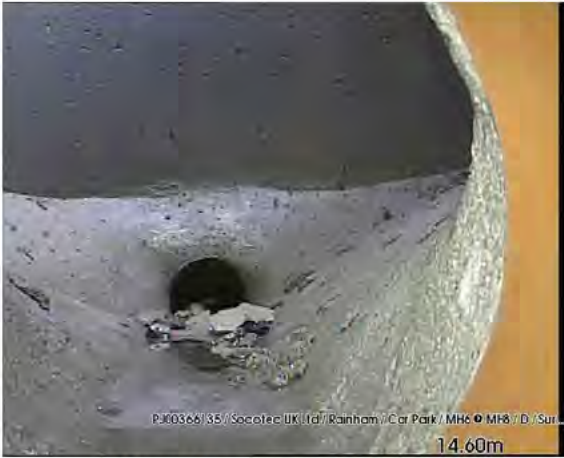
200317_1233A-Survey.jpg, 00:00:45, 14.60 m Finish node type, manhole, reference number: MH8
