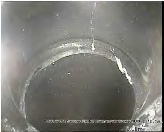
200318_1418A-Survey.jpg, 00:00:00, 0.00 m Start node type, gully, reference number: GY09
