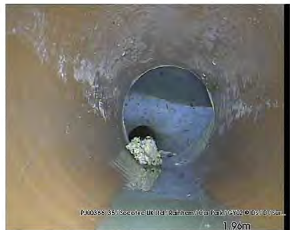
200317_1245D-Survey.jpg, 00:00:35, 1.96 m Size changes, new size(s), 150 mm high
