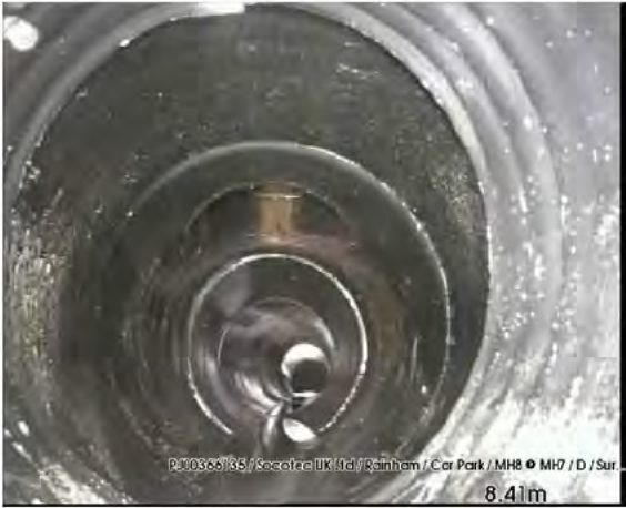
200317_1337D-Survey.jpg, 00:00:51, 8.41 m Size changes, new size(s), 225 mm high
