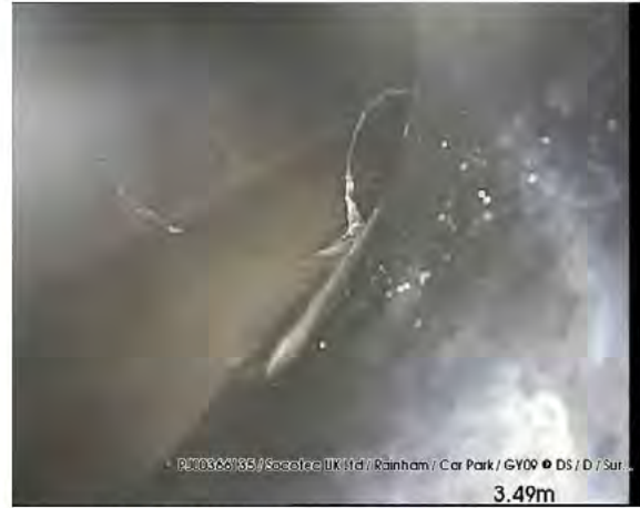
200318_1419A-Survey.jpg, 00:00:33, 3.49 m Finish node type, other special chamber, reference number: DS, reached
