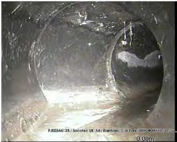
200317_1439C-Survey.jpg, 00:00:00, 0.00 m Start node type, manhole, reference number: MH9
