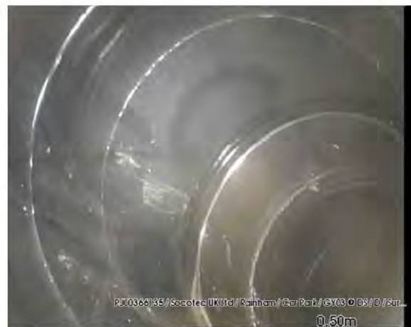
200318_1135F-Survey.jpg, 00:00:11, 0.50 m Line deviates right
