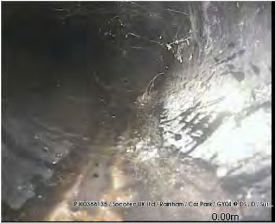
200318_1144C-Survey.jpg, 00:00:00, 0.00 m Start node type, gully, reference number: GY04
