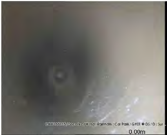
200317_1205C-Survey.jpg, 00:00:00, 0.00 m Start node type, gully, reference number: GY01
