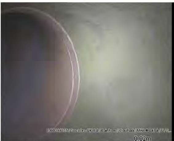
200317_1202E-Survey.jpg, 00:00:07, 0.02 m Line deviates left
