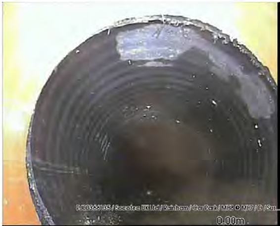
200317_1335C-Survey.jpg, 00:00:00, 0.00 m Start node type, manhole, reference number: MH8
