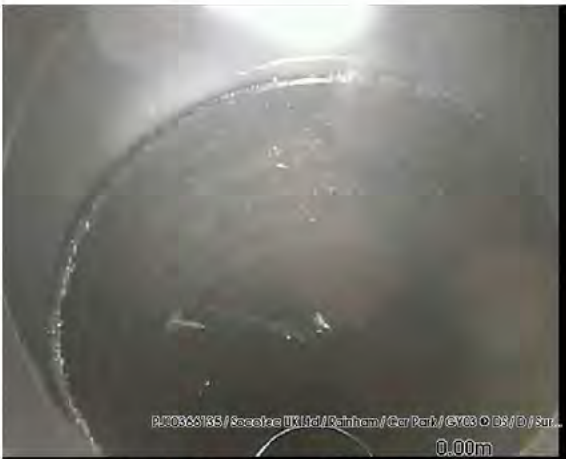
200318_1135E-Survey.jpg, 00:00:04, 0.00 m Line deviates down
