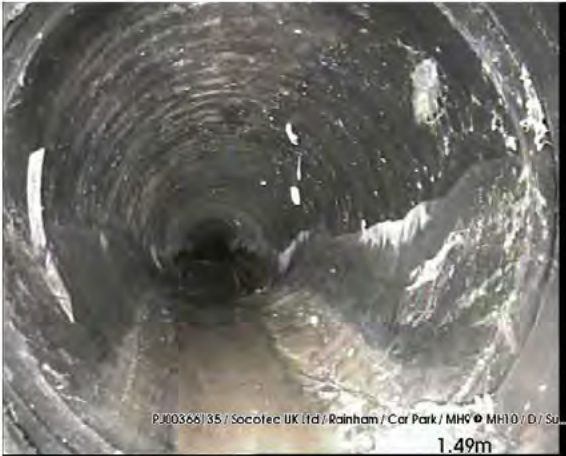
200317_1440C-Survey.jpg, 00:00:19, 1.49 m Material changes Polyvinyl chloride @REM
