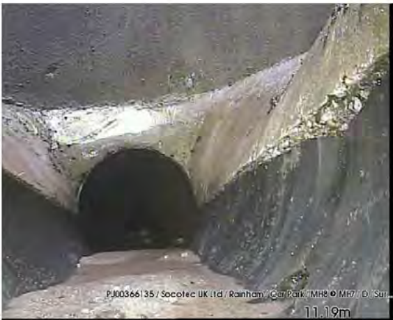
200317_1338B-Survey.jpg, 00:01:07, 11.19 m Finish node type, manhole, reference number: MH7
