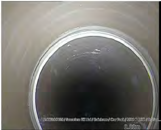
200317_1231C-Survey.jpg, 00:00:00, 0.00 m Start node type, manhole, reference number: MH6
