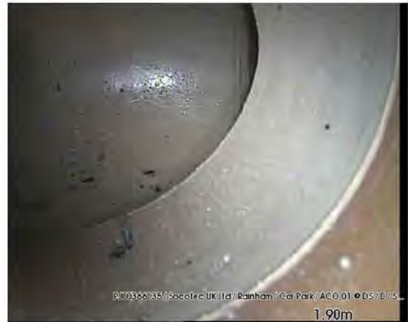
200317_1238C-Survey.jpg, 00:00:28, 1.90 m Size changes, new size(s), 150 mm high
