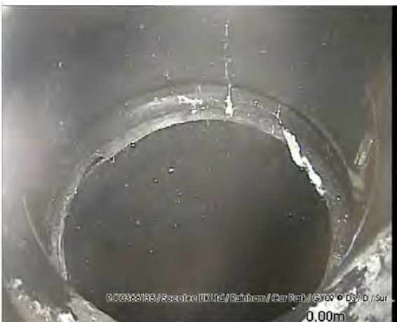
200318_1418C-Survey.jpg, 00:00:05, 0.00 m Material changes Polyvinyl chloride @REM
