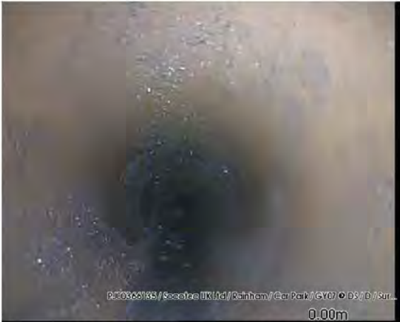
200318_1432C-Survey.jpg, 00:00:00, 0.00 m Start node type, gully, reference number: GY07
