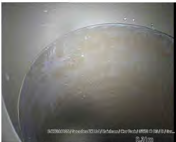
200317_1245C-Survey.jpg, 00:00:18, 0.31 m Line deviates down
