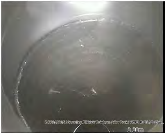
200318_1135C-Survey.jpg, 00:00:00, 0.00 m Start node type, gully, reference number: GY03
