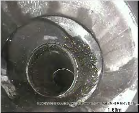
200317_1336D-Survey.jpg, 00:00:25, 1.80 m Junction, at 10 o'clock, diameter: 150 mm
