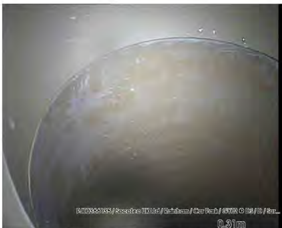
200317_1245C-Survey.jpg, 00:00:18, 0.31 m Line deviates down
