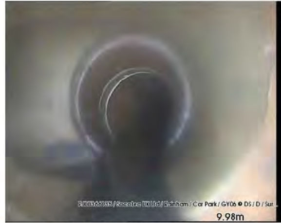
200318_1355C-Survey.jpg, 00:00:59, 9.98 m Junction, at 09 o'clock, diameter: 100 mm
