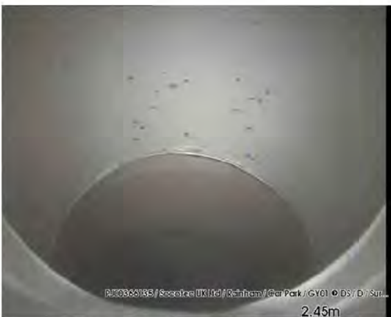
200317_1205E-Survey.jpg, 00:00:11, 2.45 m Line deviates down
