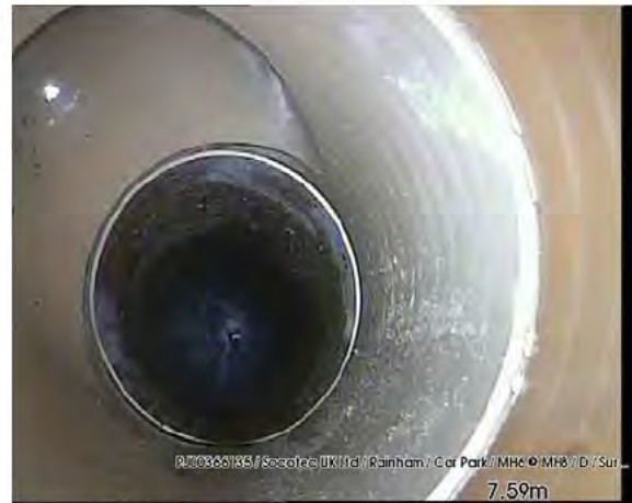
200317_1232C-Survey.jpg, 00:00:25, 7.59 m Junction, at 10 o'clock, diameter: 150 mm
