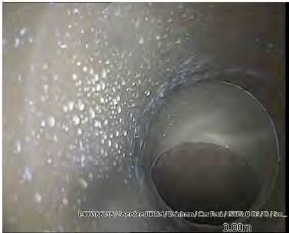
200317_1245A-Survey.jpg, 00:00:00, 0.00 m Start node type, gully, reference number: GY02
