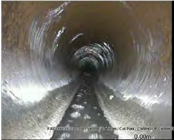
200317_1456C-Survey.jpg, 00:00:00, 0.00 m Start node type, manhole, reference number: CWMH01
