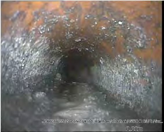
200318_1410C-Survey.jpg, 00:00:00, 0.00 m Start node type, gully, reference number: GY08
