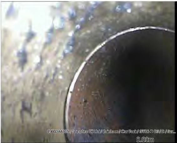
200318_1354C-Survey.jpg, 00:00:00, 0.00 m Start node type, gully, reference number: GY06
