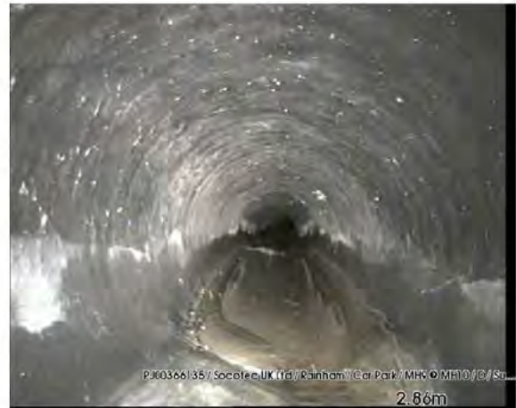
200317_1440D-Survey.jpg, 00:00:26, 2.86 m Line deviates down
