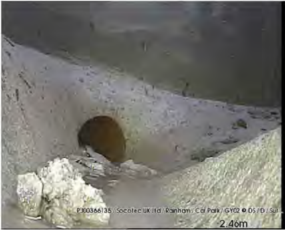
200317_1246A-Survey.jpg, 00:00:46, 2.46 m Finish node type, manhole, reference number: DS, MH8
