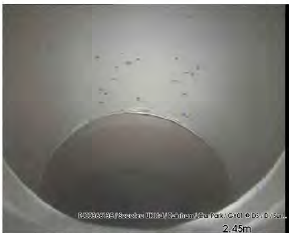
200317_1205E-Survey.jpg, 00:00:11, 2.45 m Line deviates down
