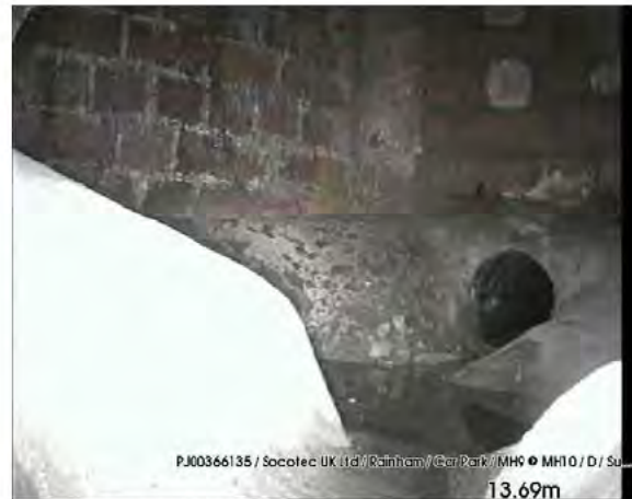
200317_1445A-Survey.jpg, 00:02:27, 13.69 m Finish node type, manhole, reference number: MH10
