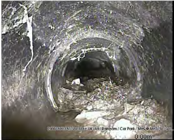
200317_1435C-Survey.jpg, 00:00:00, 0.00 m Start node type, manhole, reference number: MH9
