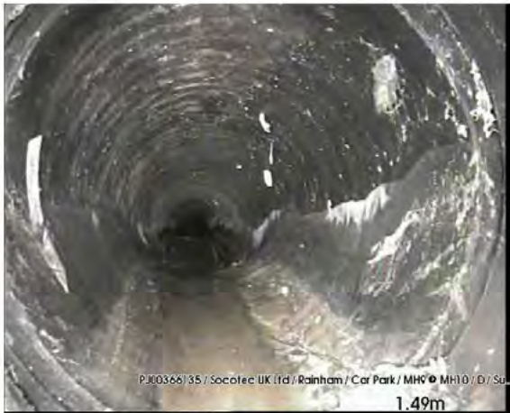
200317_1440C-Survey.jpg, 00:00:19, 1.49 m Material changes Polyvinyl chloride @REM
