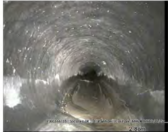
200317_1440D-Survey.jpg, 00:00:26, 2.86 m Line deviates down
