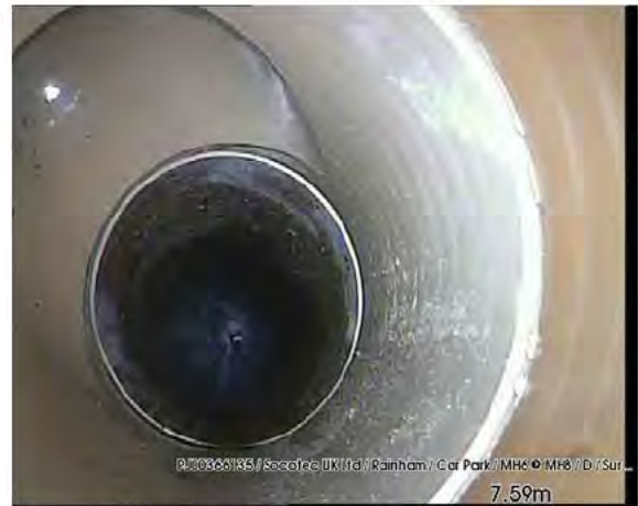
200317_1232C-Survey.jpg, 00:00:25, 7.59 m Junction, at 10 o'clock, diameter: 150 mm
