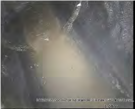
200318_1136A-Survey.jpg, 00:00:21, 1.68 m Finish node type, other special chamber, reference number: DS, REACHED
