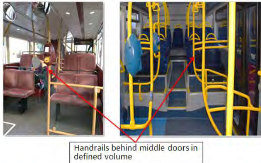
Figure 34_8: Examples of handrails positioned behind middle doors in trajectory of seated occupant that shall be identified for further assessment.
