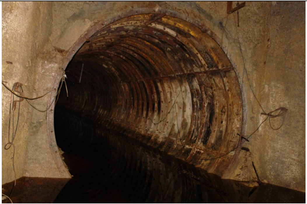
View of end of tunnel from shaft before pumping out
