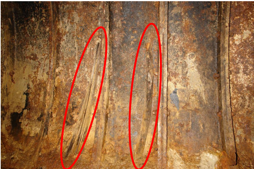
Figure 14 Timber packers for circumferential joints
