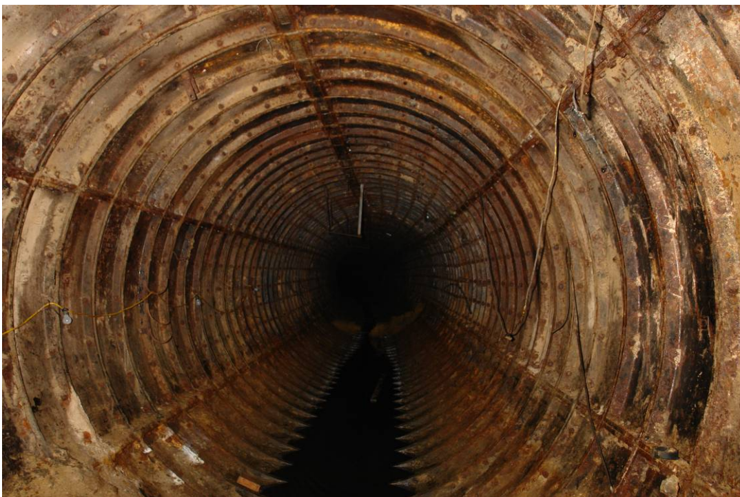
Figure 10 View of tunnel at shaft portal
