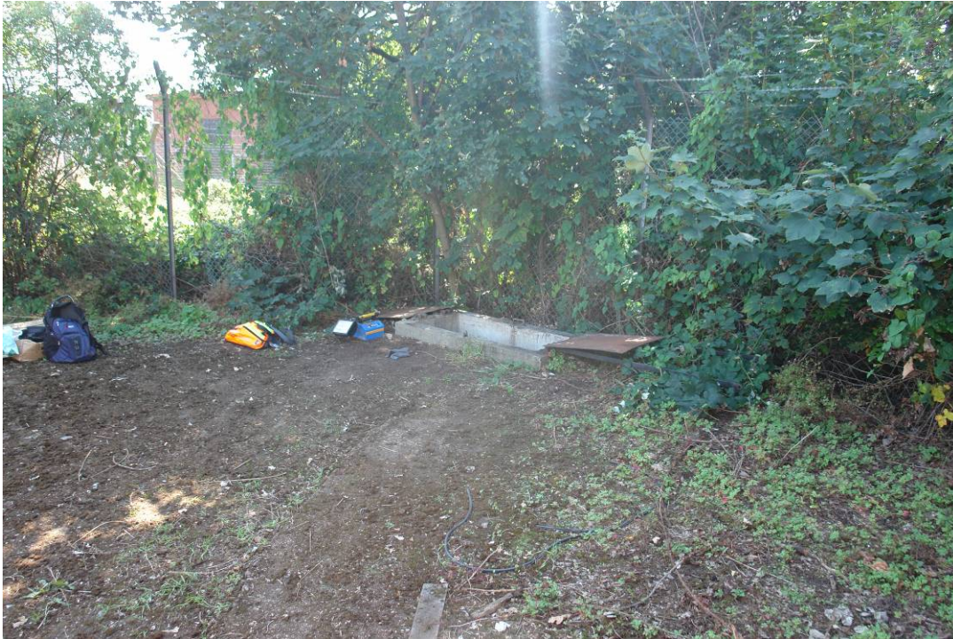
Figure 1 Soil and vegetation on top of shaft capping slab
