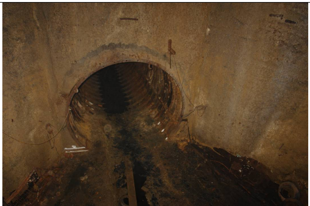
View of end of tunnel from shaft after pumping out
