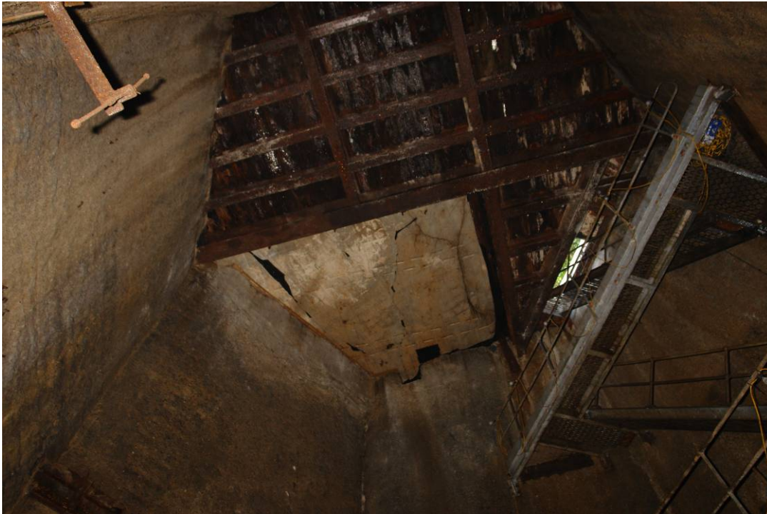
Figure 3 View of underside of slab, showing steel grillage and timber decking
