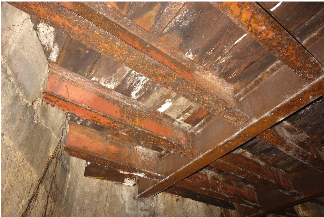
Figure 4 View of timbers and steel grillage supporting concrete slab
