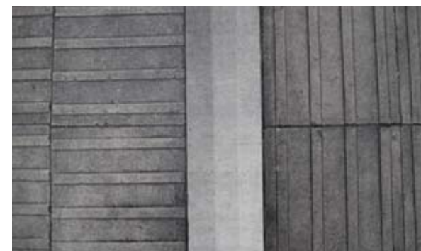
Ladder and tramline with raised delineator
