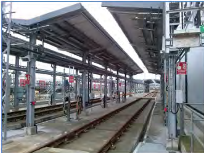
Winterisation Facility Constructed at Neasden Depot for Sanding and De-icing refill for S-Stock
