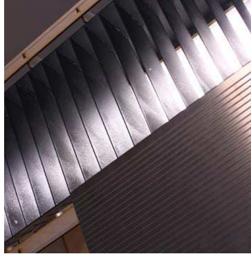
Contrast between illuminated black louvre and diffuse light emitter - potential for photosensitive risk to be evaluated at prototype stage
