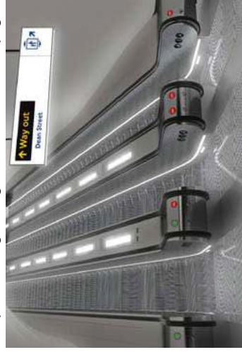
Deep-recessing of original SPL-502 deck uplight would compromise soft-edge illumination of vault
