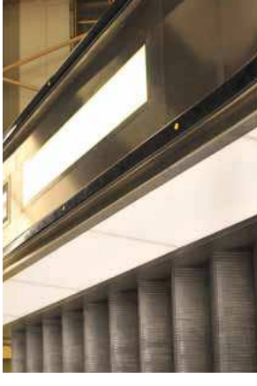
Design intent photo of backlit LED uplight in a mock-up position and in relation to the backlit balustrade
