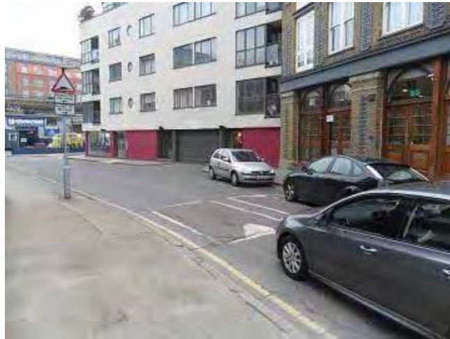
Photograph 4: Speed cushions on Union Street
