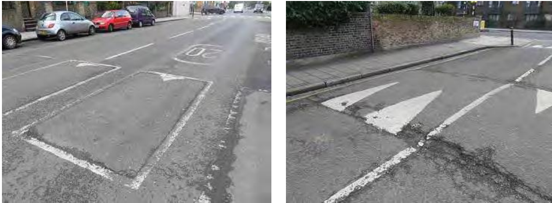
Photograph 2 (L-R): Speed cushions on Liverpool Road and speed hump on Furlong Road
