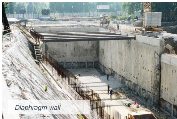
Diaphragm wall construction
