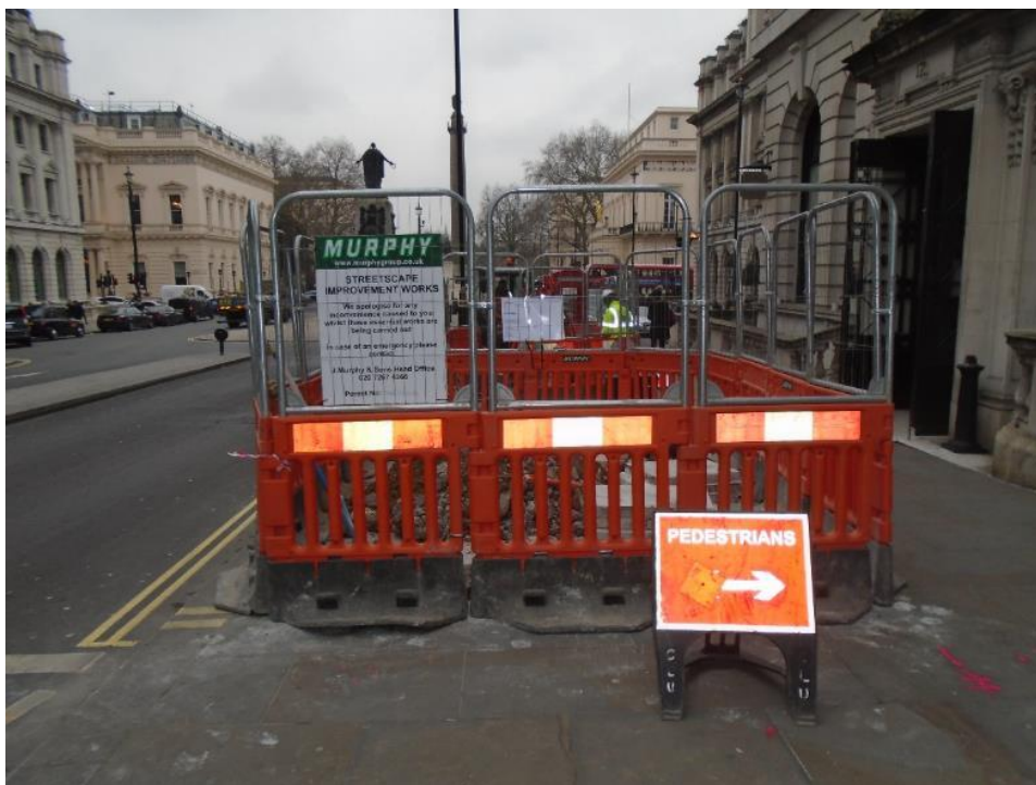
Figure 3-2: Photo of Strongwall Barrier in use to secure a works area
