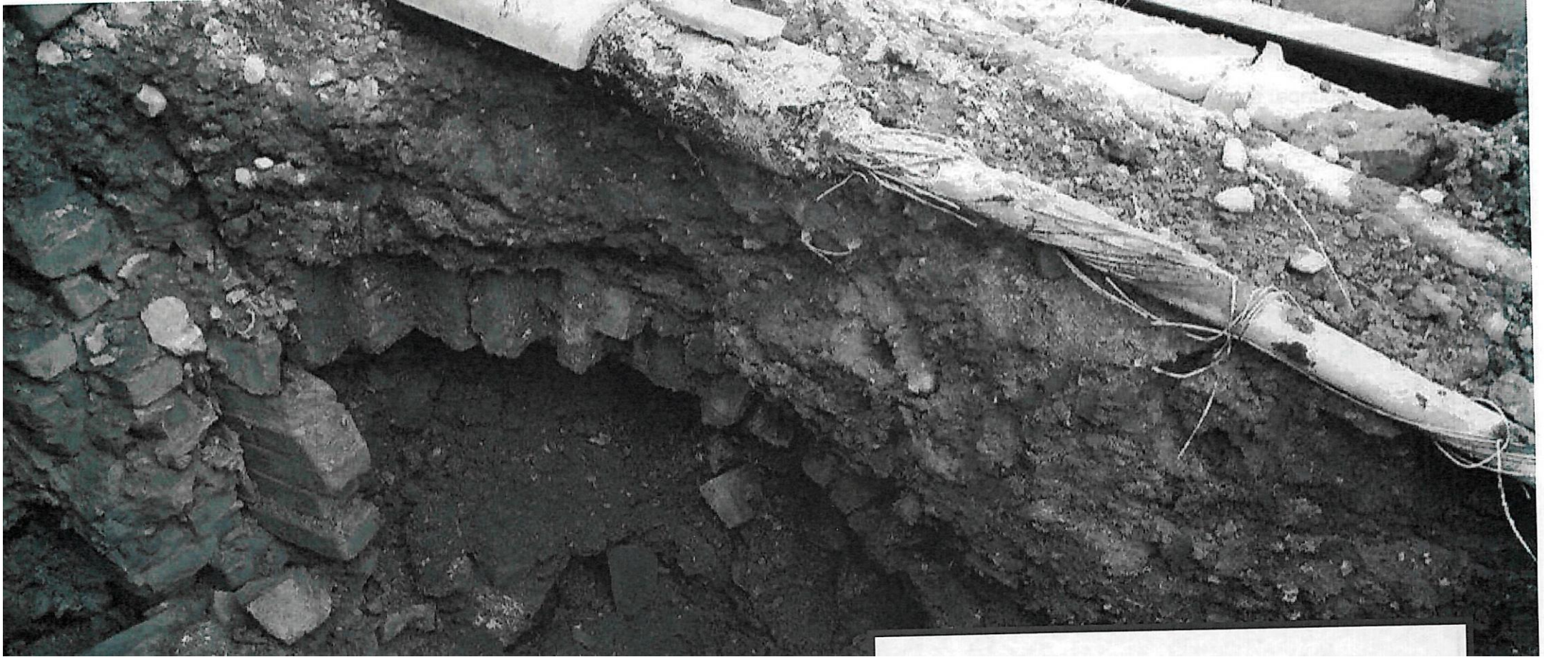
Appendix B - 6.2.2 Early Warning Notice C422-EWN-00532 Photograph 2 - Unsuitable backfill within redundant cellar
