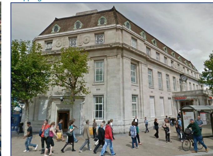
Figure 6.2: Listed Building to the front of Centre Court Shopping Centre
