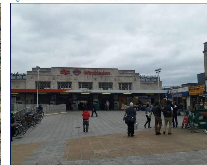
Figure 6.4: Entrance to Wimbledon Station
