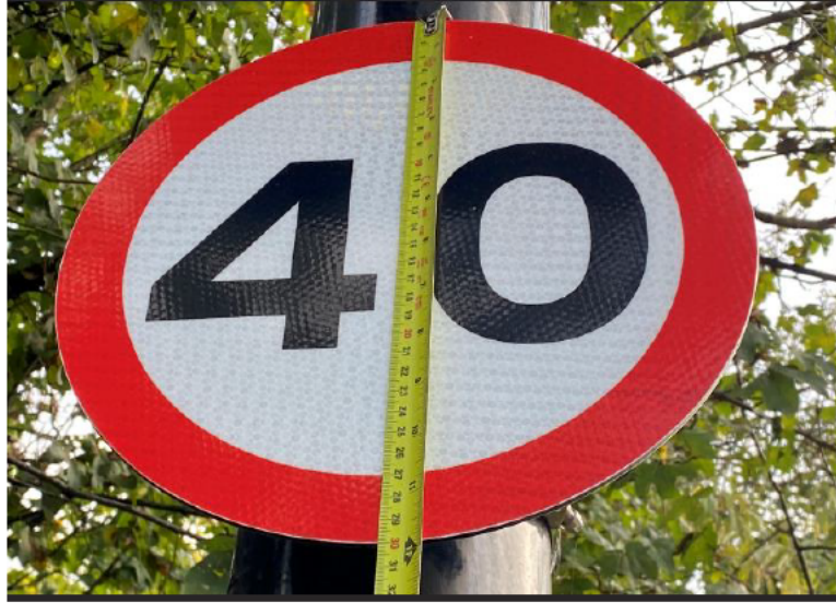
Figure 2 – Size of the new 40mph repeaters (300mm)
