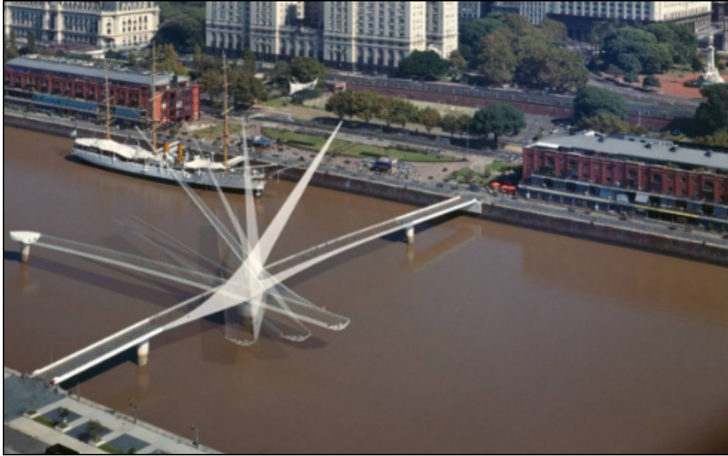
Figure 3-3 Puente de la Mujer swing bridge in Buenos Aires
